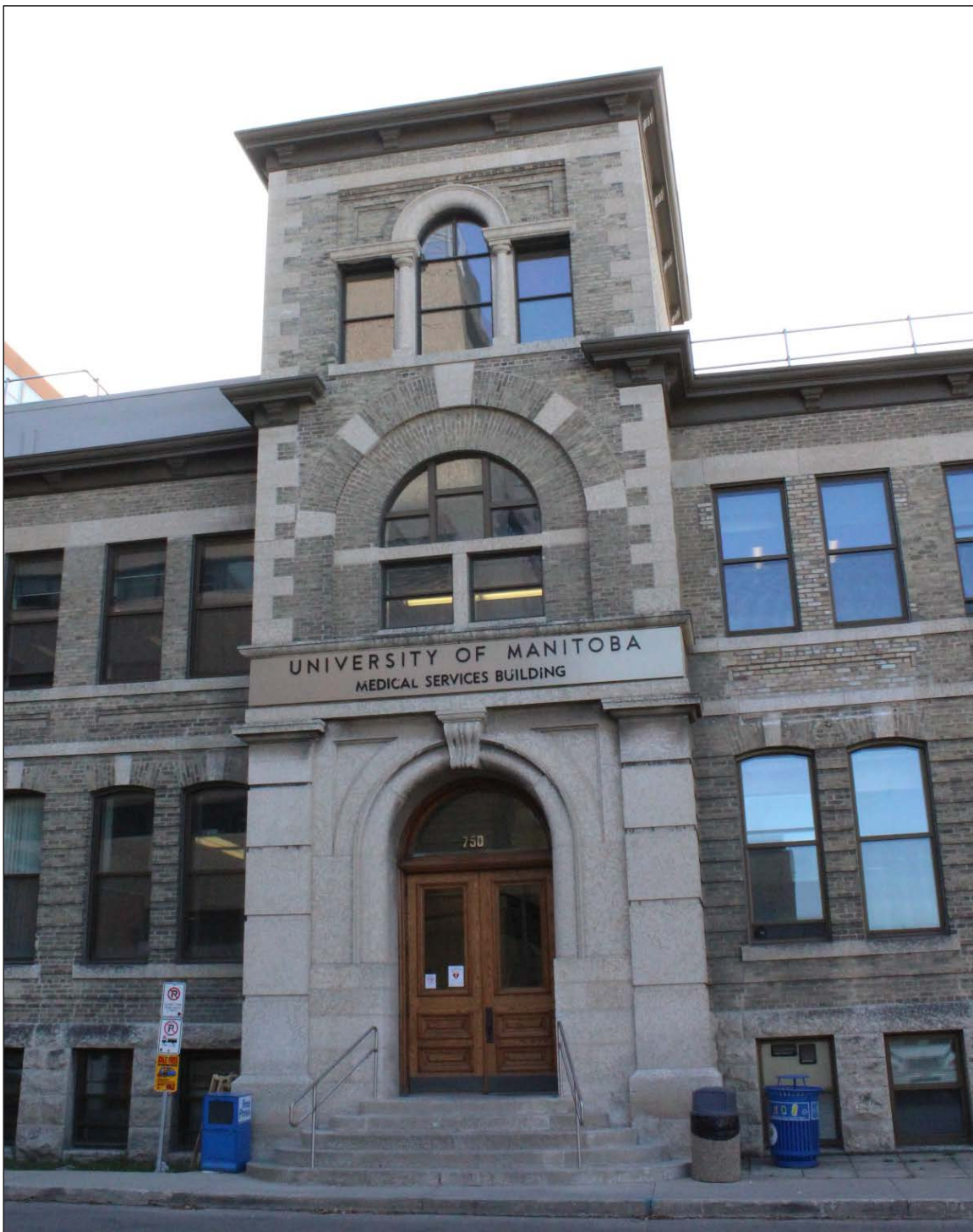
Plate 13 – Manitoba Medical College (University of Manitoba Faculty of Medicine Building), 750 Bannatyne Avenue, detail of main (north) entrance, 2017. (M. Peterson, 2017.)
