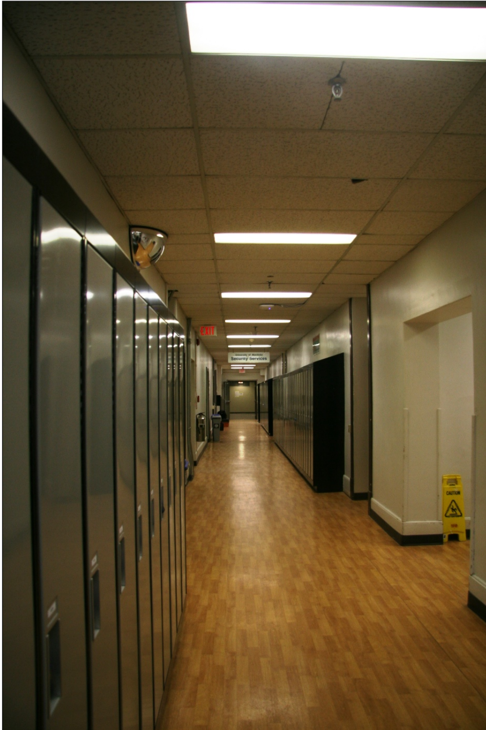
Plate 20 – Manitoba Medical College (University of Manitoba Faculty of Medicine Building), 750 Bannatyne Avenue, typical renovated space (ground floor) with new floors, acoustic ceiling and fluorescent lighting, 2018. ( T. Andreoglou, 2018. )
