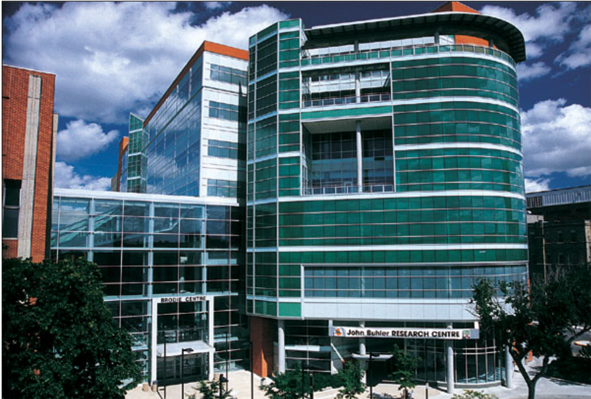
Plate 28 – Brodie Centre, 727 Bannatyne Avenue, no date. (Reproduced from M.D. Steele Construction Company website, http://www.mdsteele.mb.ca/projects.asp?cat=5 .)
