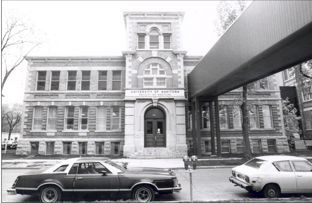
Plate 21 – Manitoba Medical College (University of Manitoba Faculty of Medicine Building), 750 Bannatyne Avenue, with overhead walkway, 1978. ( City of Winnipeg. )
