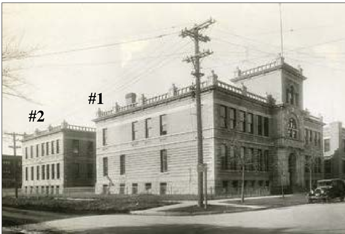
Plate 8 – Manitoba Medical College, Bannatyne Avenue, front (north) and east façades, 1930. This picture shows the original building and the 1909 (#1) and 1913 (#2) additions. (University of Manitoba Faculty of Medicine Archives, “MMC 1930”, UMFMA 0007C in https://archivescanada.accesstomemory.ca .)
