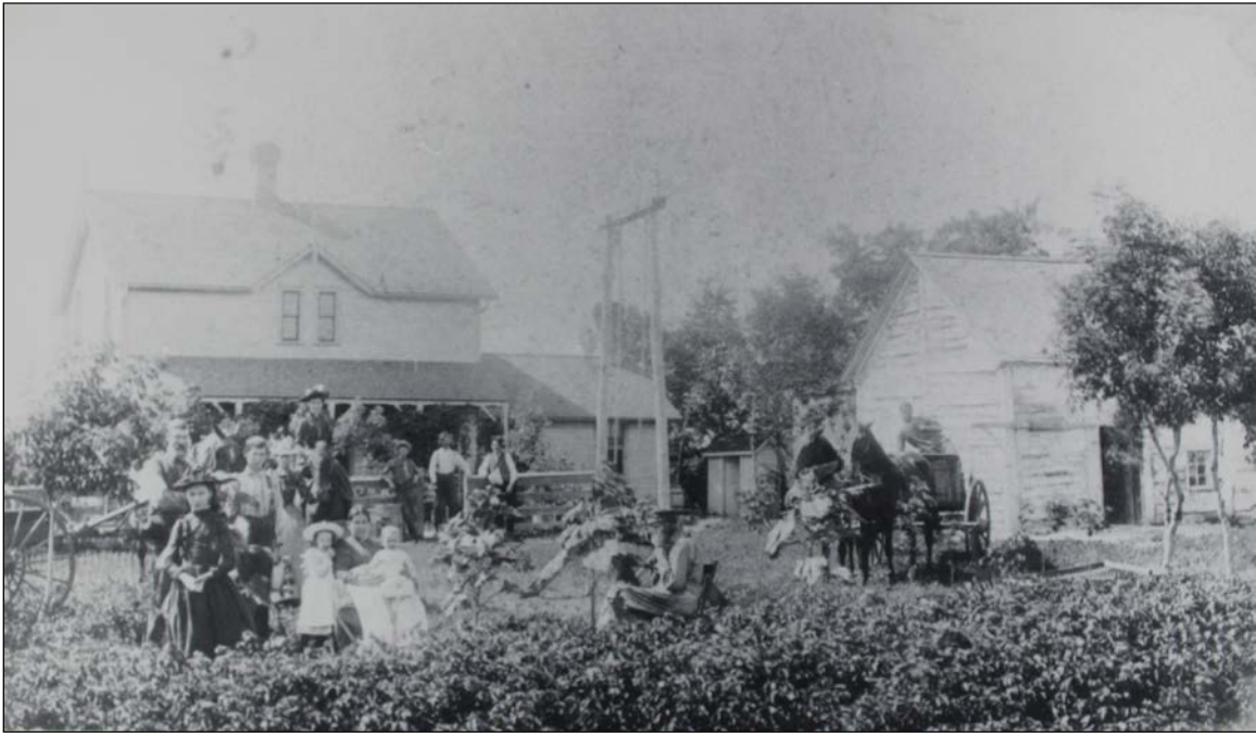
Plate 14 – The John Smith family poses for this photograph in front of their farmhouse and barn in ca.1903. A large, prosperous venture, the land was bought in 1904 by the City of Winnipeg, reportedly for nearly $40,000, to create City Park, today’s Assiniboine Park. ( Archives of Manitoba, “Agriculture- Farms- 88,” N15653. )
