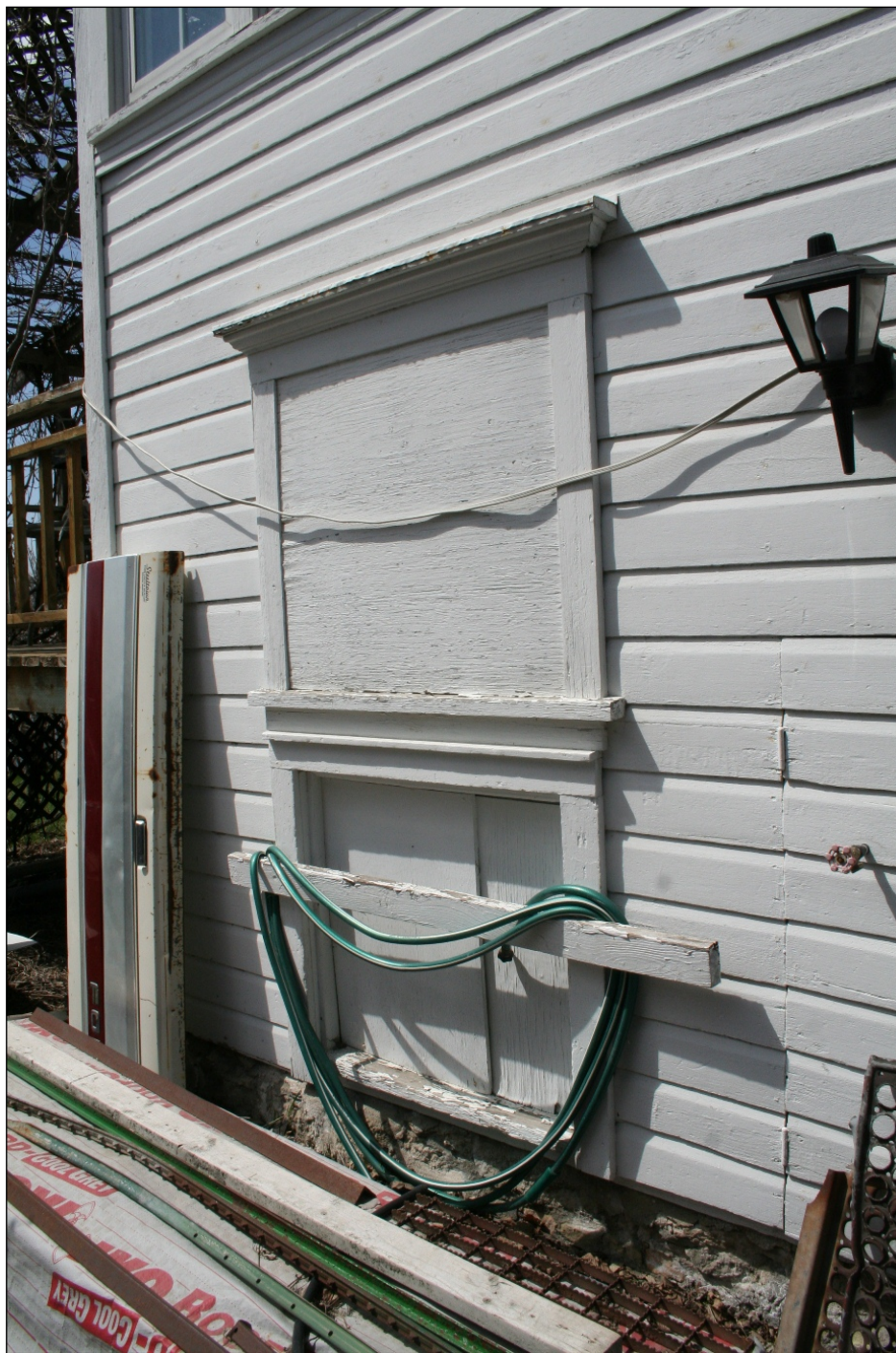
Plate 12 – Ellis Boarding House, 43 Boyle Street, two-part opening in east end, 2013. ( M. Peterson, 2013. )
