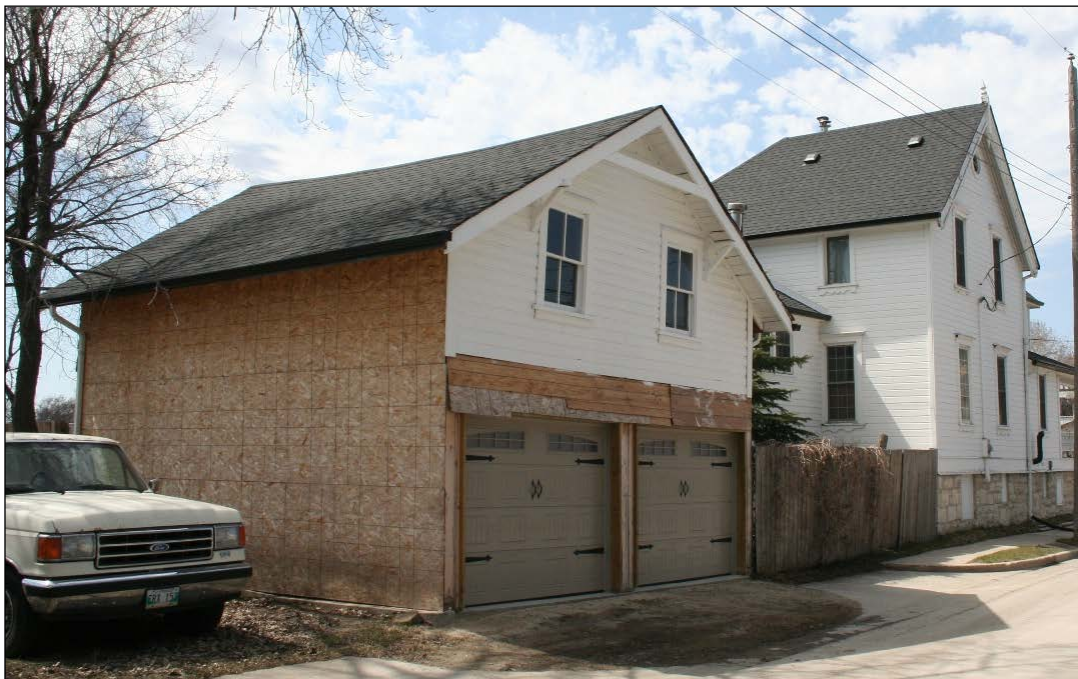
Plate 7 – Ellis Boarding House, 43 Boyle Street, carriage house in 1977 (top) and 2013 (bottom). ( City of Winnipeg, 1977 & M. Peterson, 2013. )
