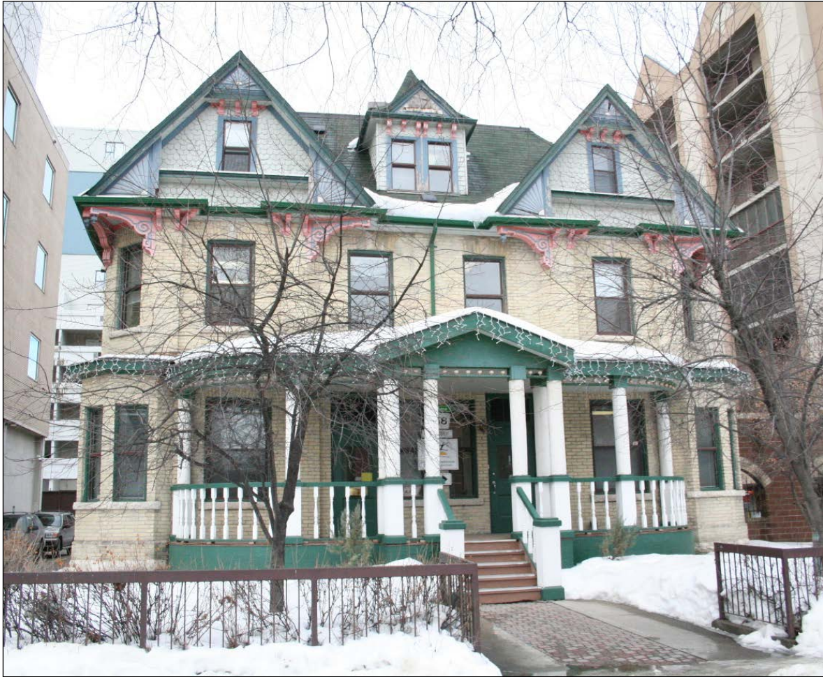
Plate 5 – Duplex, 368-70 Edmonton Street, front (east) façade, 2007; built in 1901, architect Johann Schwab. (M. Peterson, 2007.)
