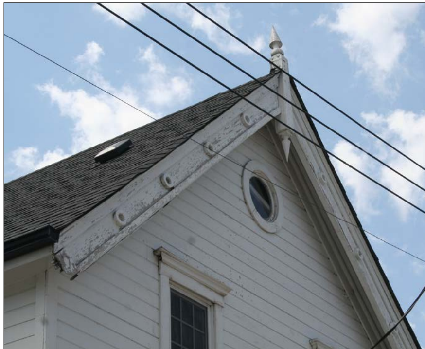
Plate 9 – Ellis Boarding House, 43 Boyle Street, detail of north façade, 2013. ( M. Peterson, 2013. )
