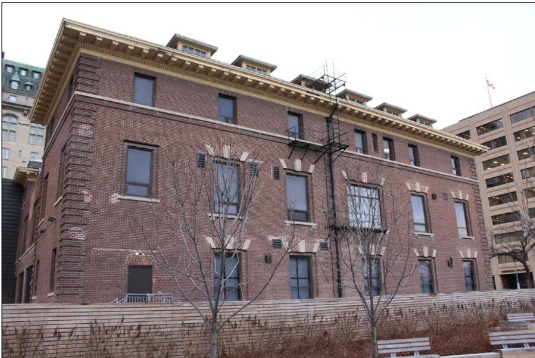
Plate 14 – Manitoba Club, 194 Broadway, east façade, 2016. (M. Peterson, 2016.)
