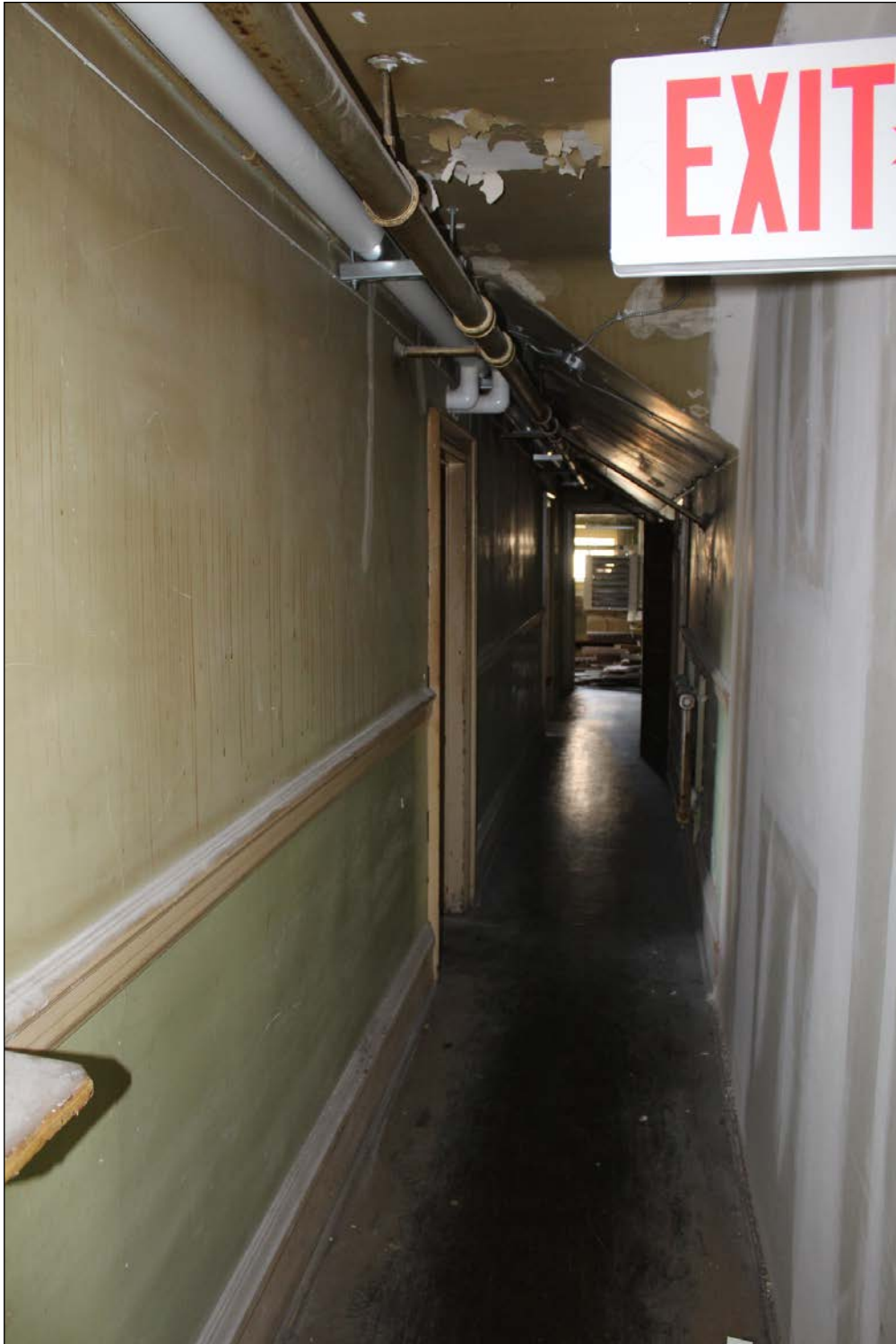
Plate 32 – Manitoba Club, 194 Broadway, attic hallway, 2017. ( M. Peterson, 2017. )
