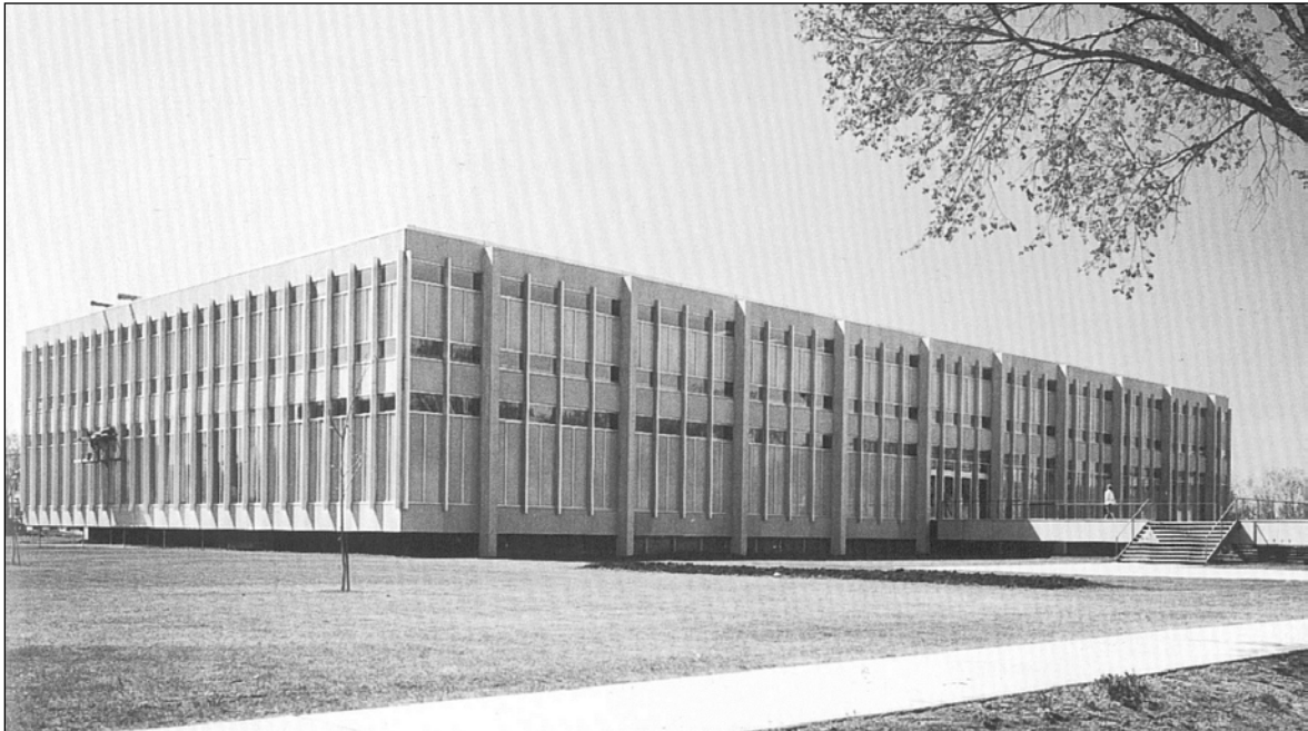
Plate 27 – Two views of the J.A. Russell Building, 83 Dafoe Road. The top (north façade) is from 1957 and the bottom (north and east façades) is from 1962. (Top: Reproduced from Smith Carter website, http://www.smithcarter.com/our_history/1947_1960/ ; and bottom: University of Manitoba Archives, Henry Kalen Photograph, 249D5.2-31.)
