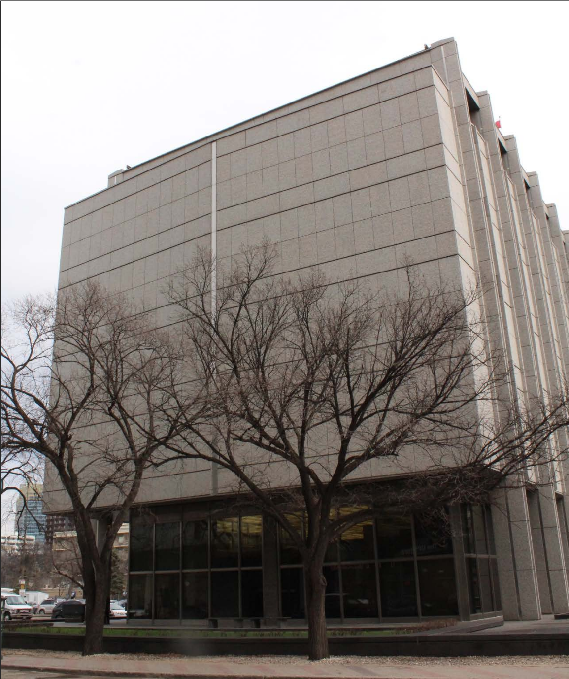
Plate 13 – Monarch Life Building, 333 Broadway, west façade, 2016. (M. Peterson, 2016.)
