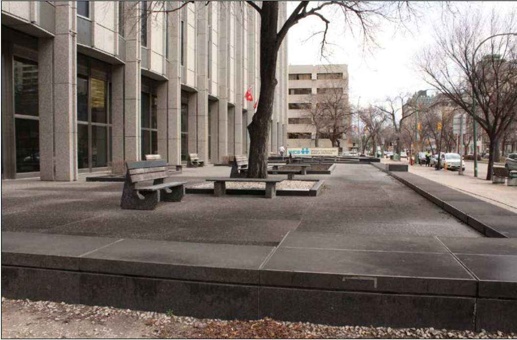
Plate 9 – Monarch Life Building, 333 Broadway, pedestal and ground floor, front (south) façade, 2016. ( M. Peterson, 2016. )
