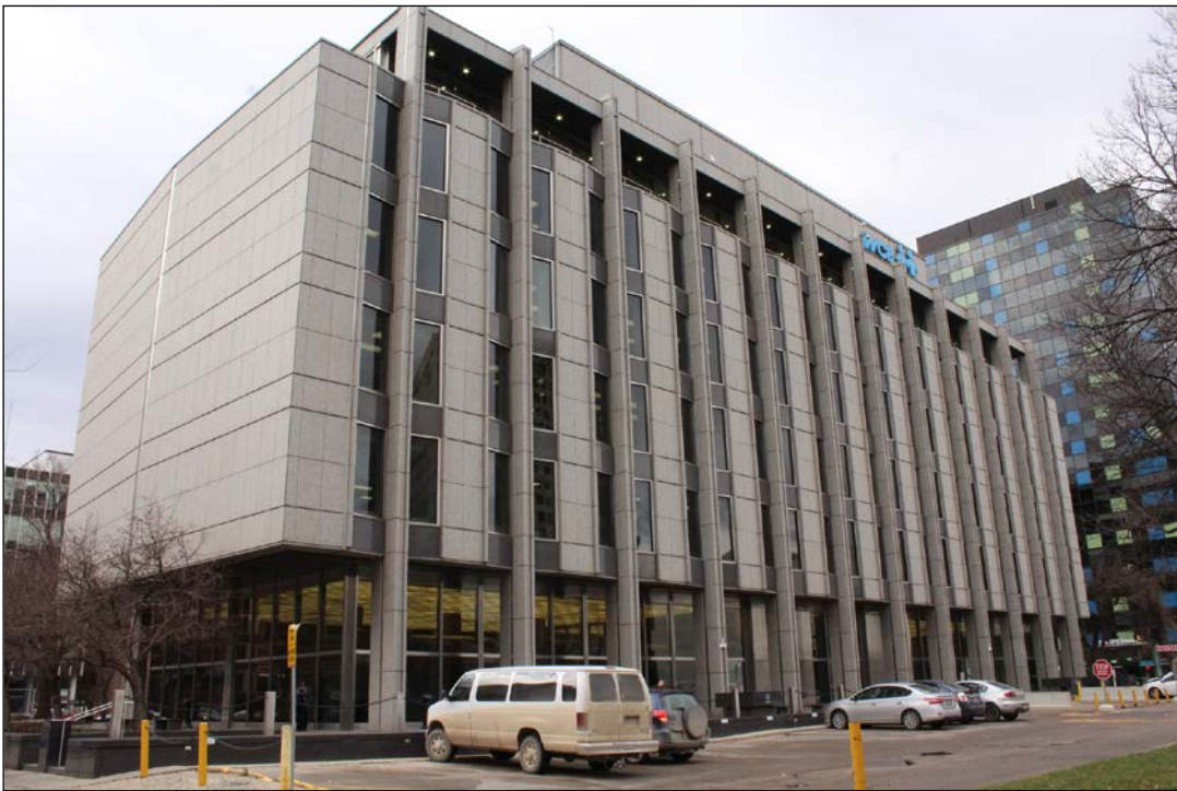
Plate 12 – Monarch Life Building, 333 Broadway, north and east façades, 2016. ( M. Peterson, 2016. )
