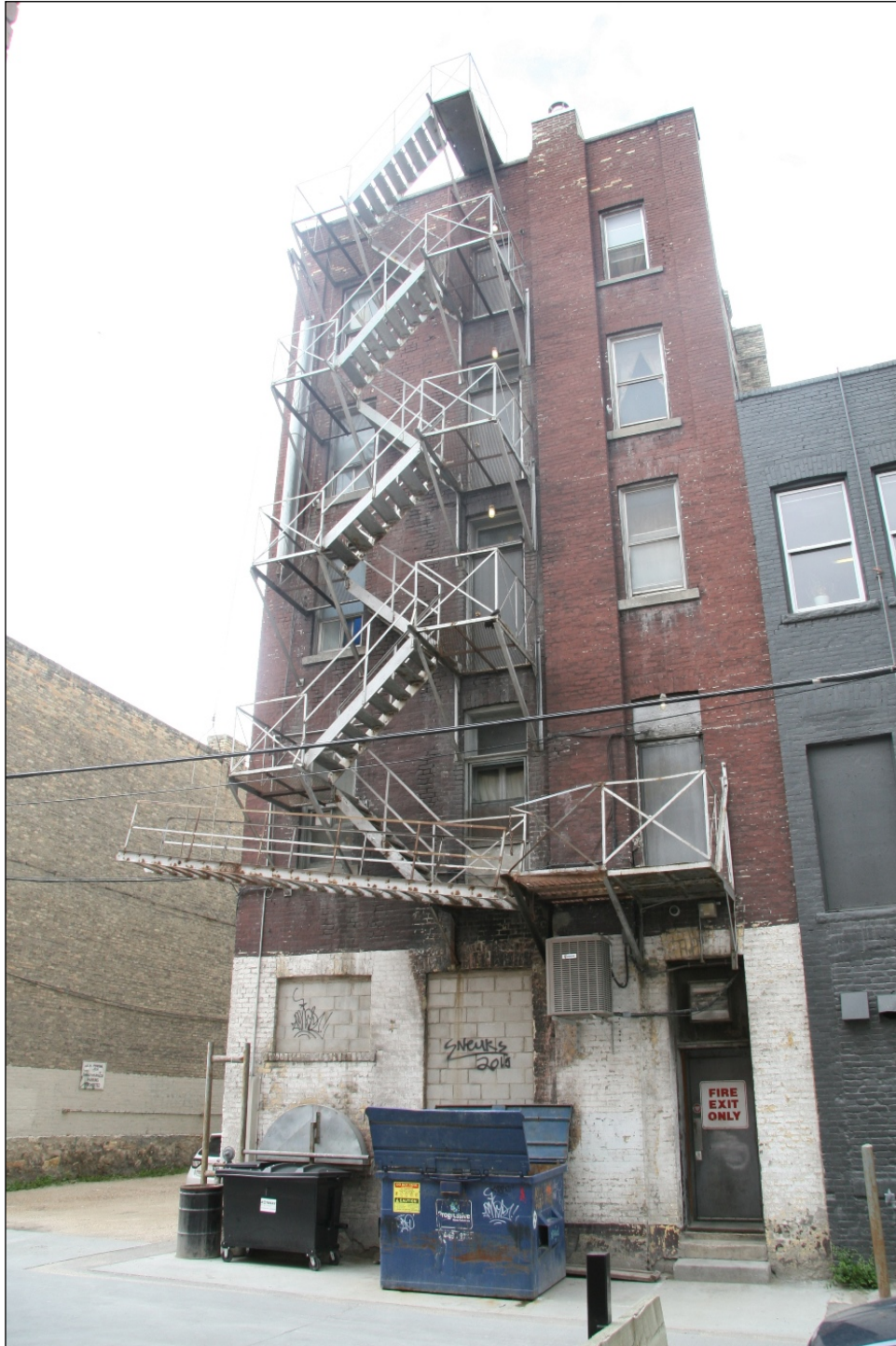
Plate 11 – Garrick Hotel, 287 Garry Street, rear (east) façade, 2015. ( M. Peterson, 2015. )
