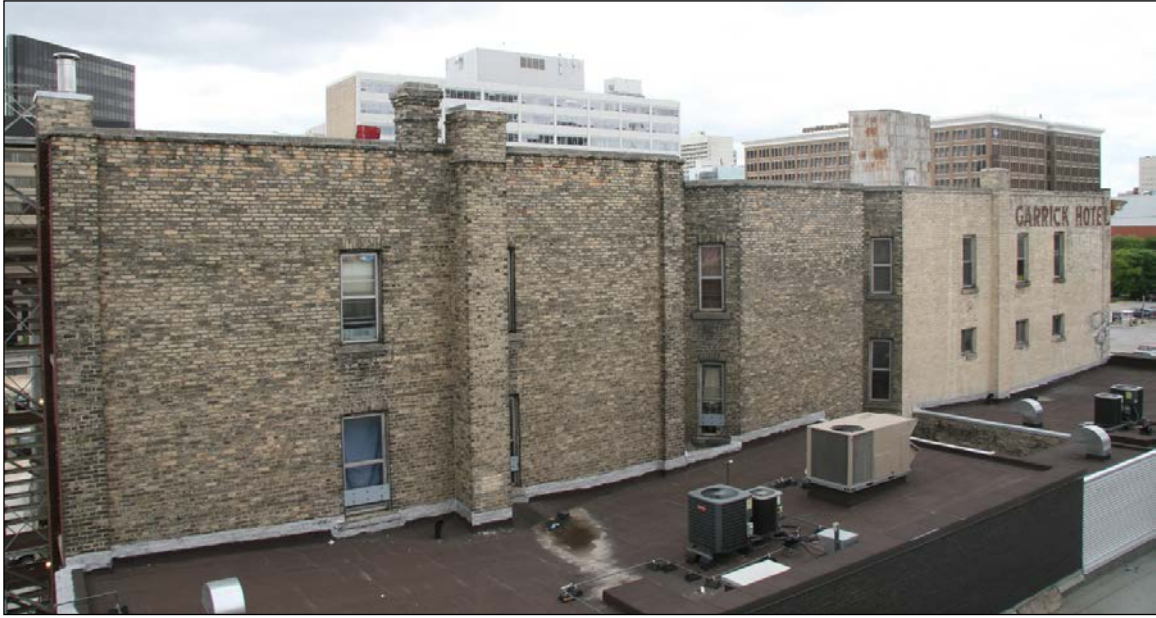
Plate 12 – Garrick Hotel, 287 Garry Street, north façade, 2015. ( M. Peterson, 2015. )
