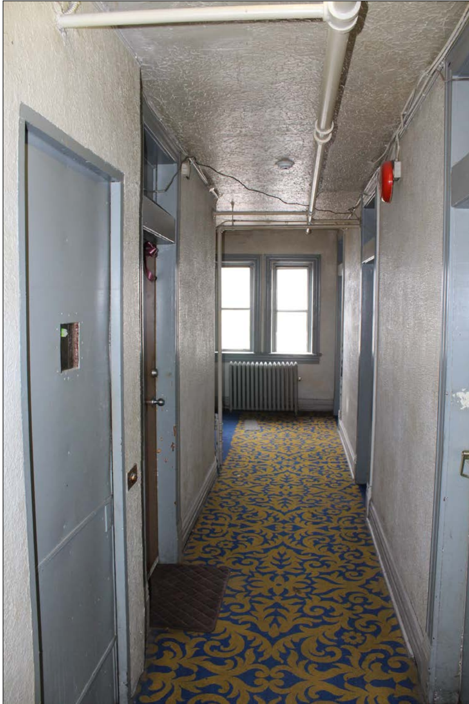
Plate 14 – Garrick Hotel, 287 Garry Street, 5 th floor hallway, 2016. ( M. Peterson, 2016. )
