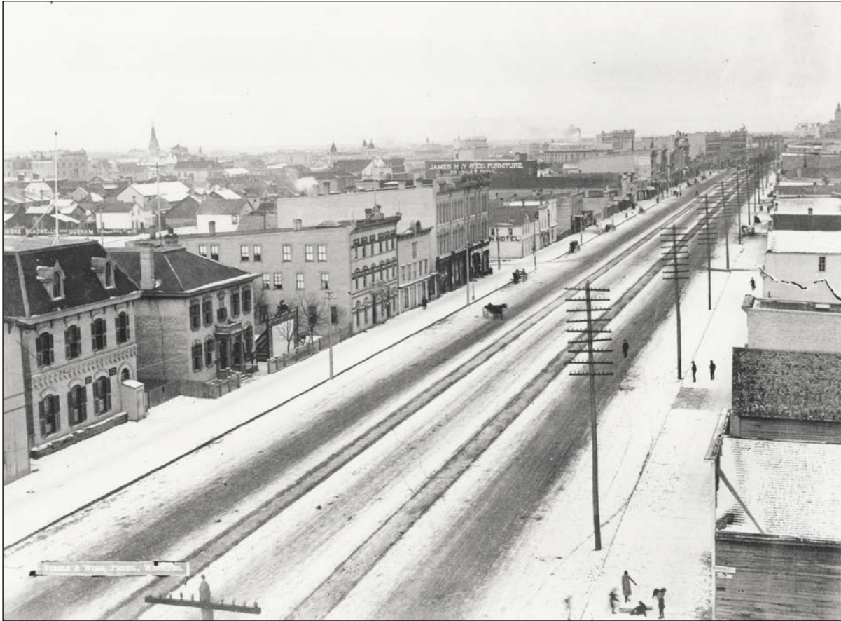
Plate 1 – West side of Main Street between York and St. Mary streets, 1892. Note the lack of empty lots as far as the eye can see north. Buildings on the left from south to north are: Dominion Lands Office; Trust and Loan Co. of Canada; Winnipeg Hotel (still standing); Dominion Hotel; Commercial Hotel (still standing) and the Fortune Block (still standing). ( Archives of Manitoba, Victor Acker Collection- 2, N842. )
