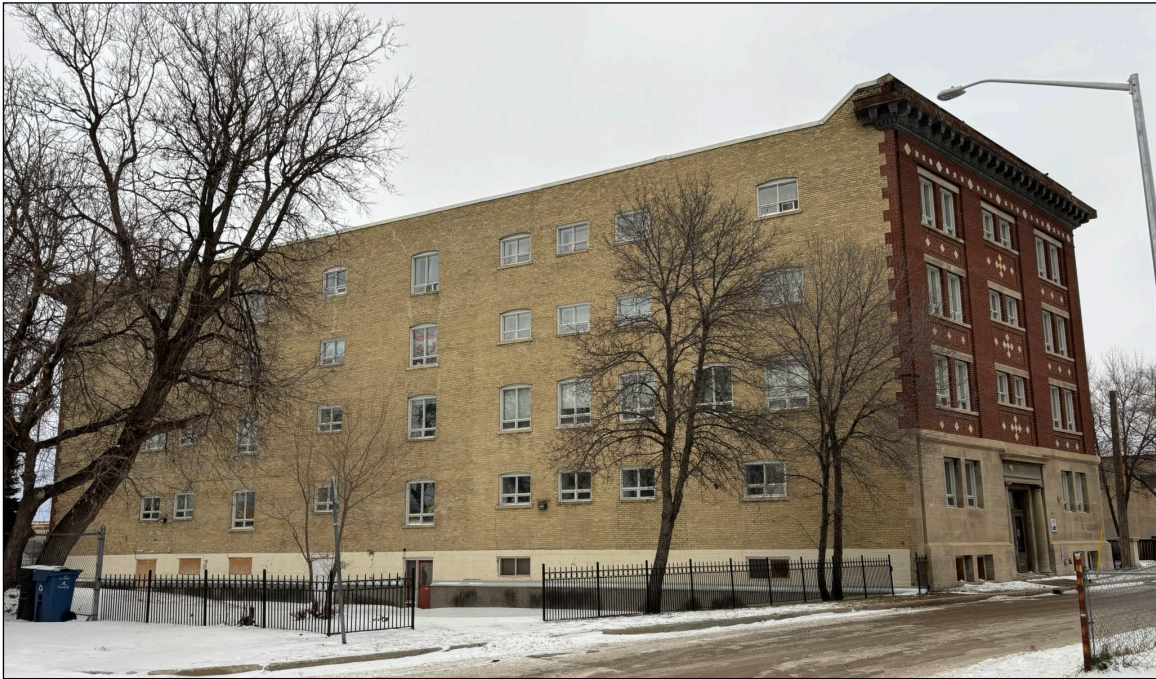
Plate 11 – Turner & Walker Block, 425 Henry Avenue, front (south) and west façades, 2024. ( M. Peterson, 2024. )
