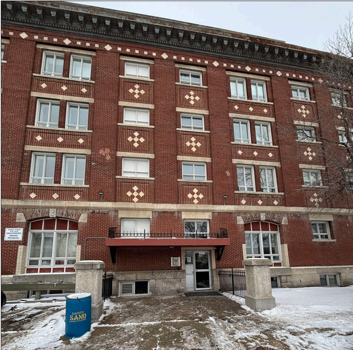
Plate 13 – Turner & Walker Block, 425 Henry Avenue, east façade entrance, 2024. (M. Peterson, 2024.)
