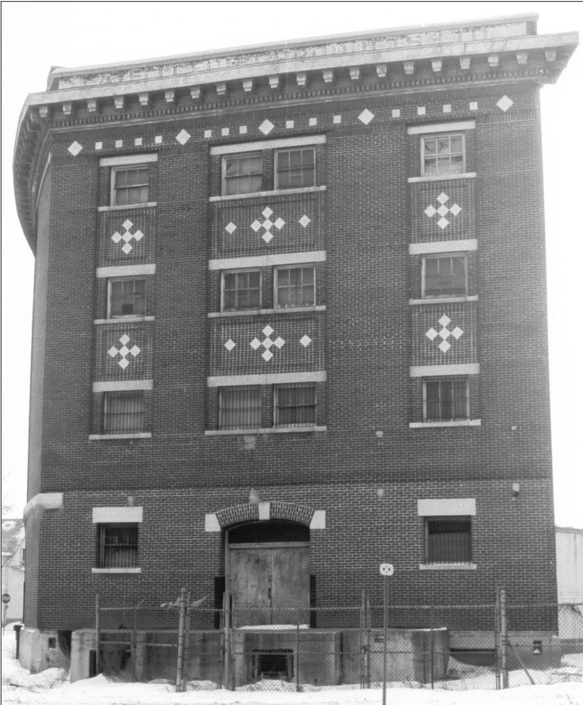
Plate 17 – Turner-Walker Block, 425 Henry Avenue, rear (north) façade, 1987. ( M. Peterson, 1987. )
