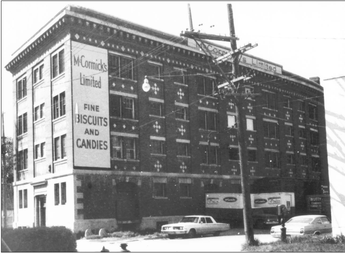
Plate 16 – Turner and Walker Block, 425 Henry Avenue, front (south) and east façades, 1969. ( Archives of Manitoba, Architectural Survey. )
