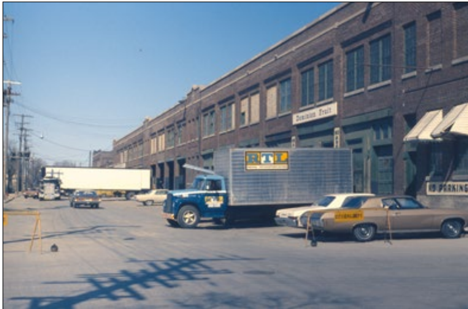
Plate 46 – Midland Fruit Warehouse, 401-433 Ross Avenue, south façade, 1973. ( Historical Buildings and Resources Committee Collection. )
