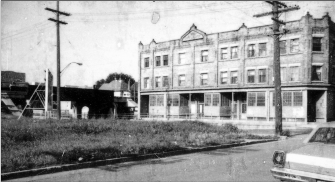
Plate 41 – Orris Block, 926-930 Sherbrook Street with Midland Railway subway to the left, ca.1961. When the subway was approved in 1911, 4.9 metres were demolished from the south end of the block, which was owned by the railway. ( Historical Buildings and Resources Committee Collection. )
