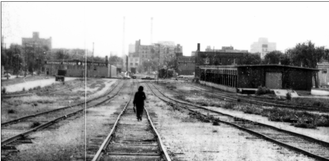
Plate 38 – Midland Railway Building, 200 Isabel Street (north and west façades), looking east from Sherbrook Street down the right-of-way, ca. 1965. ( Historical Buildings and Resources Committee Collection. )
