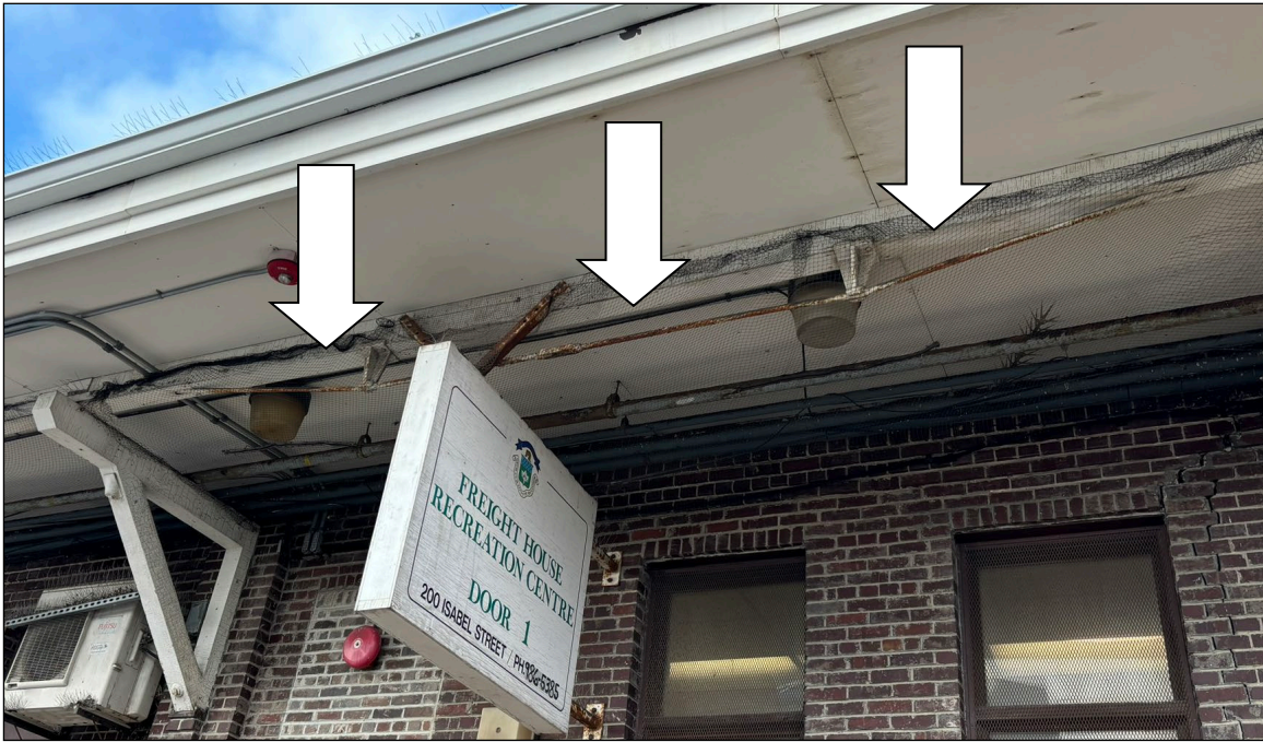
Plate 18 – Midland Railway Building, 200 Isabel Street, metal turnbuckle bracing, south façade, 2024. (M. Peterson, 2024.)
