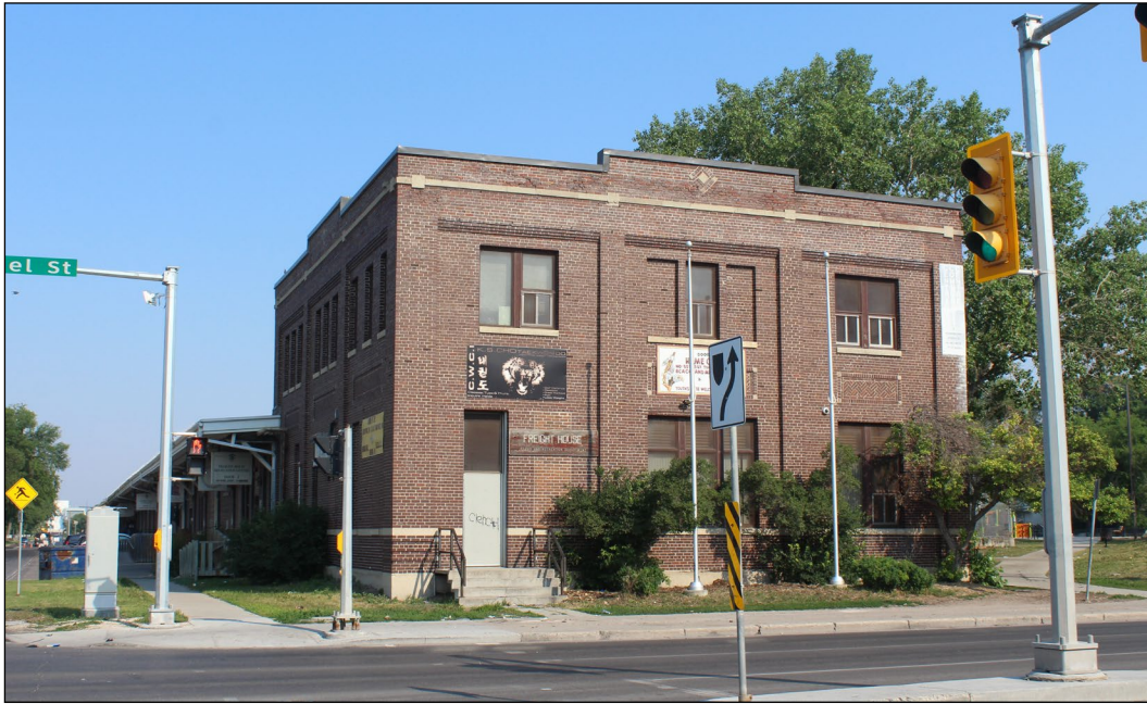
Plate 12 – Midland Railway Building, 200 Isabel Street, front (east) and south façades, 2021. ( M. Peterson, 2021. )
