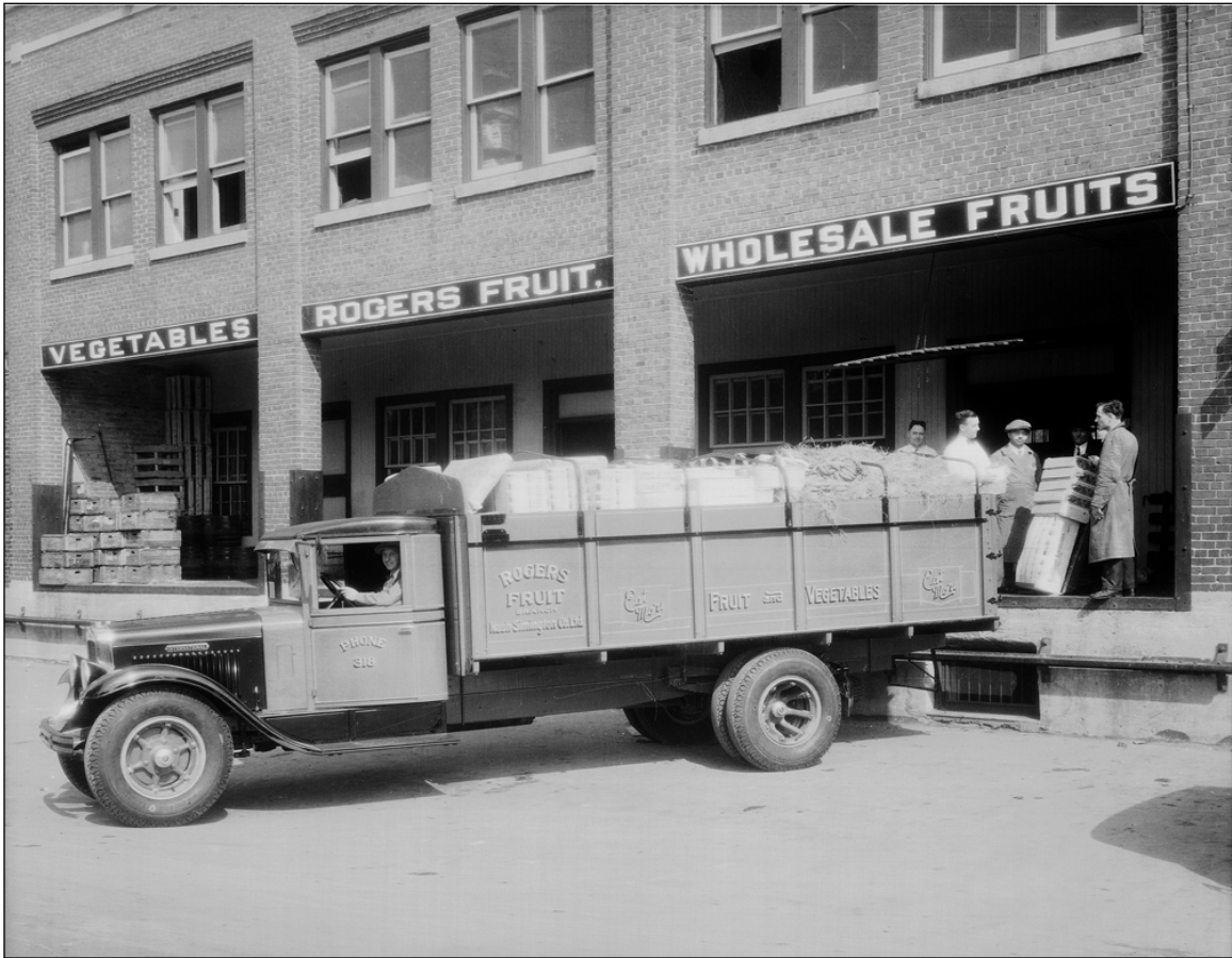
Plate 44 – Midland Fruit Warehouse, 401-433 Ross Avenue, south façade, ca.1935. ( Historical Buildings and Resources Committee Collection. )
