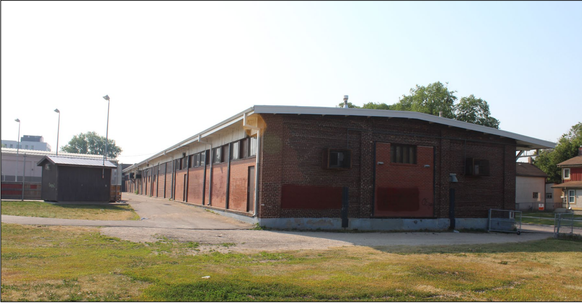
Plate 21 – Midland Railway Building, 200 Isabel Street, north and west façades, 2021. ( M. Peterson, 2021. )
