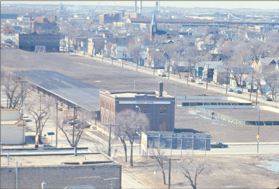
Plate 39 – Image of the Midland Railway Building from the east, date unknown. Although there is no signage, the outdoor hockey rinks to the north of the building suggest it is being converted into a community centre, ca.1974. ( Historical Buildings and Resources Committee Collection. )
