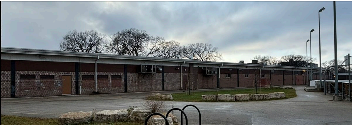
Plate 22 – Midland Railway Building, 200 Isabel Street, west end of the north façade, showing the bricking in of the original openings, 2024. ( M. Peterson, 2024. )
