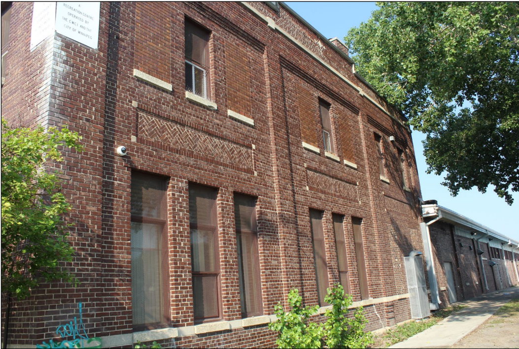
Plate 14 – Midland Railway Building, 200 Isabel Street, north façade, 2021. (M. Peterson, 2021.)
