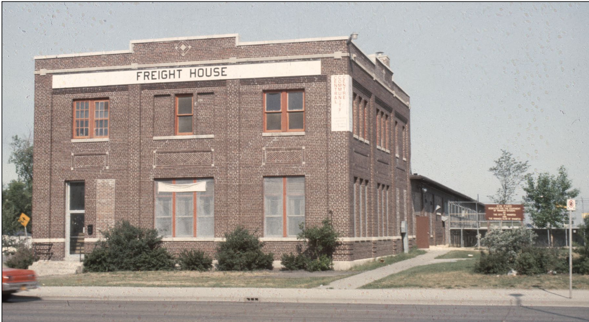
Plate 47 – Freight House – Central Community Centre, 200 Isabel Street, front (east) and north façades, ca.1975. (Historical Buildings and Resources Committee Collection.)
