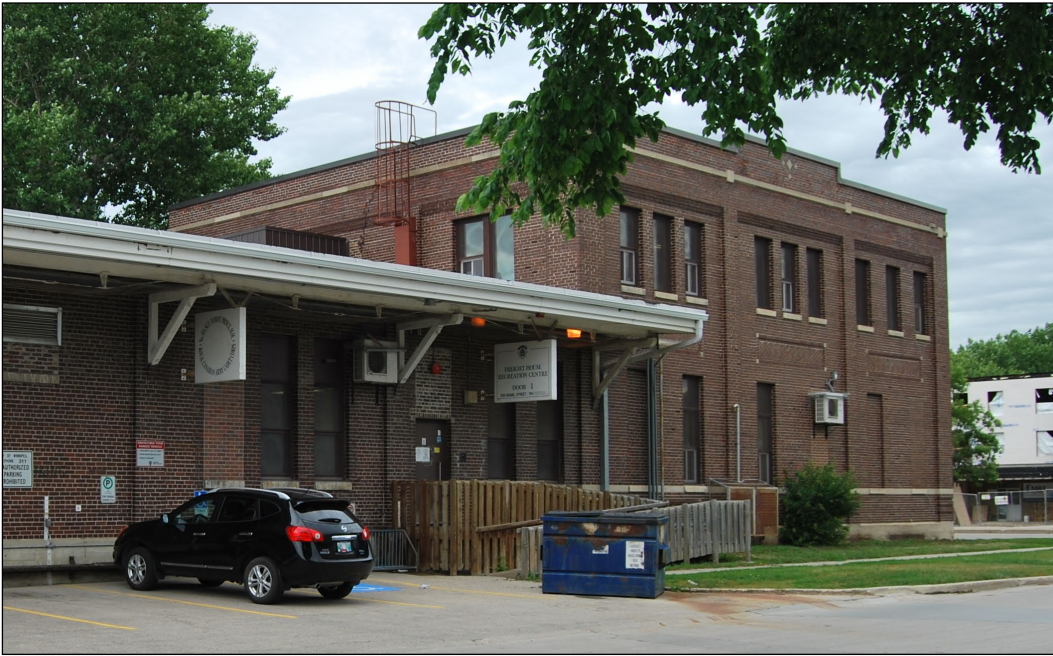
Plate 16 – Midland Railway Building, 200 Isabel Street, south and west façades of two-storey portion, 2013. ( M. Peterson, 2013. )
