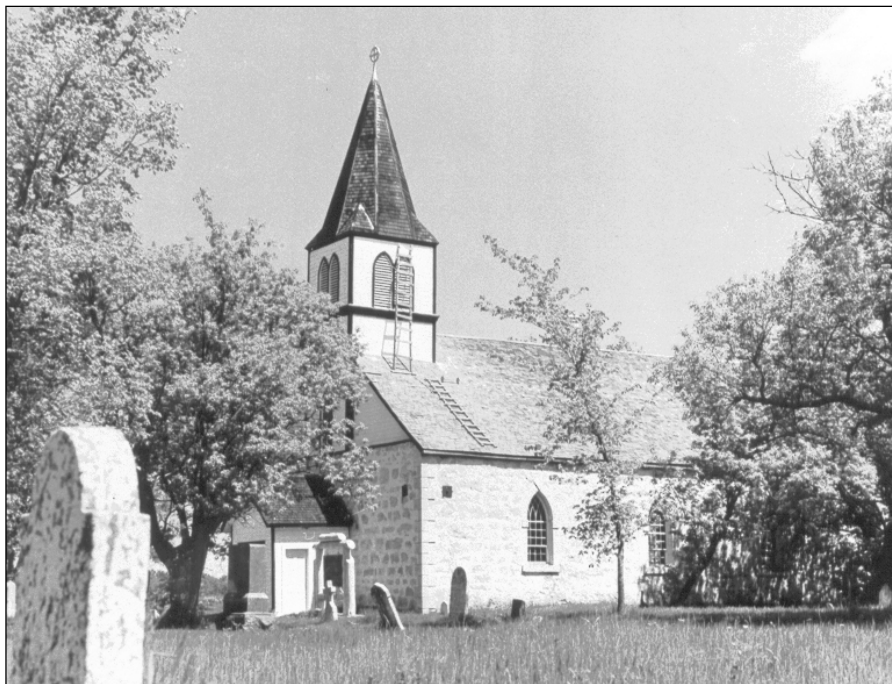
Plate 5 – St. Peter's Dynevor Anglican Church, St. Clements Municipality; built 1852-53, Duncan McRae and William Cockran, architects, Duncan McRae stonemason. ( Photo courtesy of the Western Canada Pictorial Index, Negative 52-1568. )
