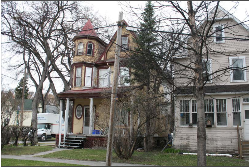
Front (south) and east façades, 2009
