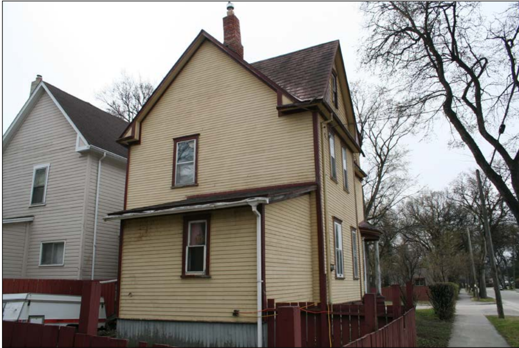
Rear (north) and west façades, 2009
