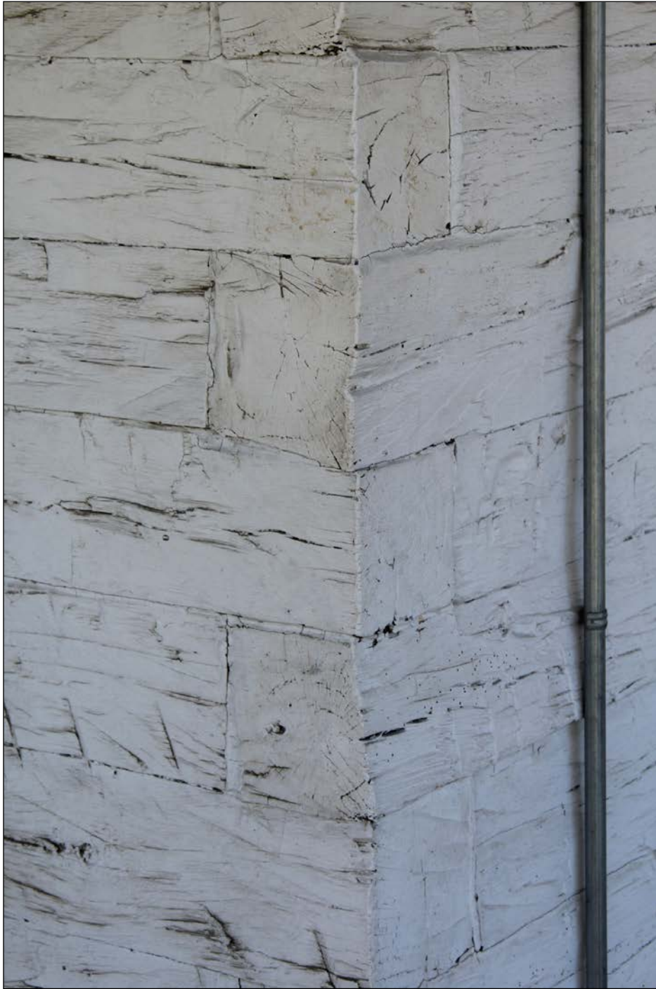
Plate 9 – Seven Oaks Museum, John and Mary Inkster House, 50 Mac Street, southwest corner, showing dovetail joints, 2020. ( M. Peterson, 2020. )
