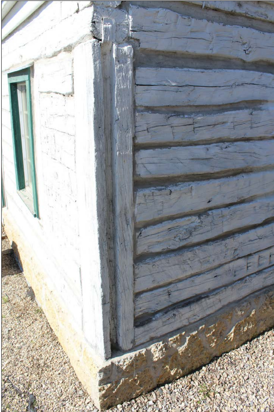
Plate 7 – First John and Mary Inkster House, 50 Mac Street, northeast corner, Red River frame construction, 2020. ( M. Peterson, 2020. )
