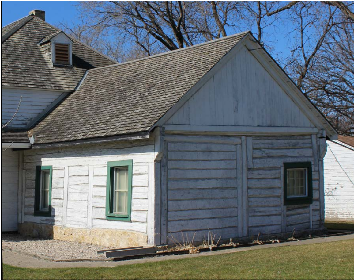
Plate 8 –John and Mary Inkster House, 50 Mac Street, north end kitchen, Red River frame construction, 2020. ( M. Peterson, 2020. )
