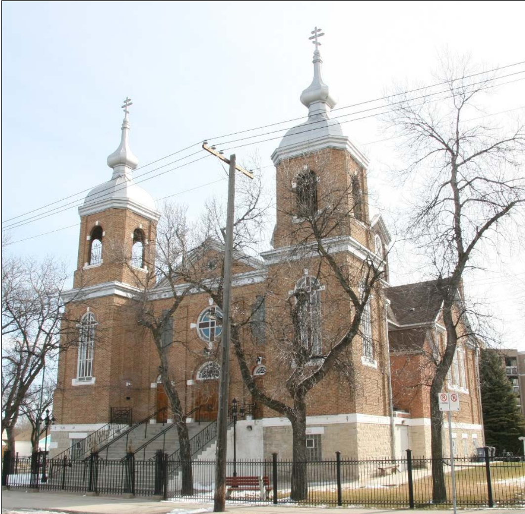
Plate 3 – St. Mary the Protectress Ukrainian Orthodox Sobor, 820 Burrows Avenue, front and south façades, 2016; built between 1925 and 1951. ( M. Peterson, 2016. )
