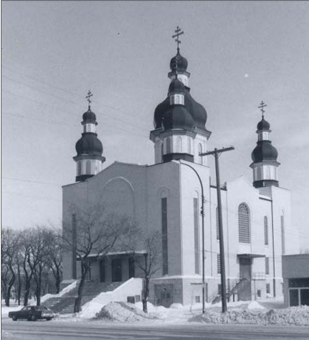
Plate 8 – Holy Trinity Ukrainian Orthodox Metropolitan Cathedral, 1175 Main Street, 1978, showing the front (west) façade prior to the addition of the mosaic. ( City of Winnipeg. )
