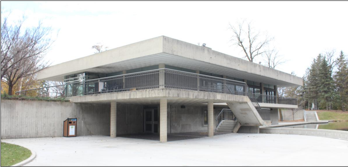
Plate 24 – Peguis Pavilion, Kildonan Park, 2015 Main Street, east and north façades, 2022. ( M. Peterson, 2022. )
