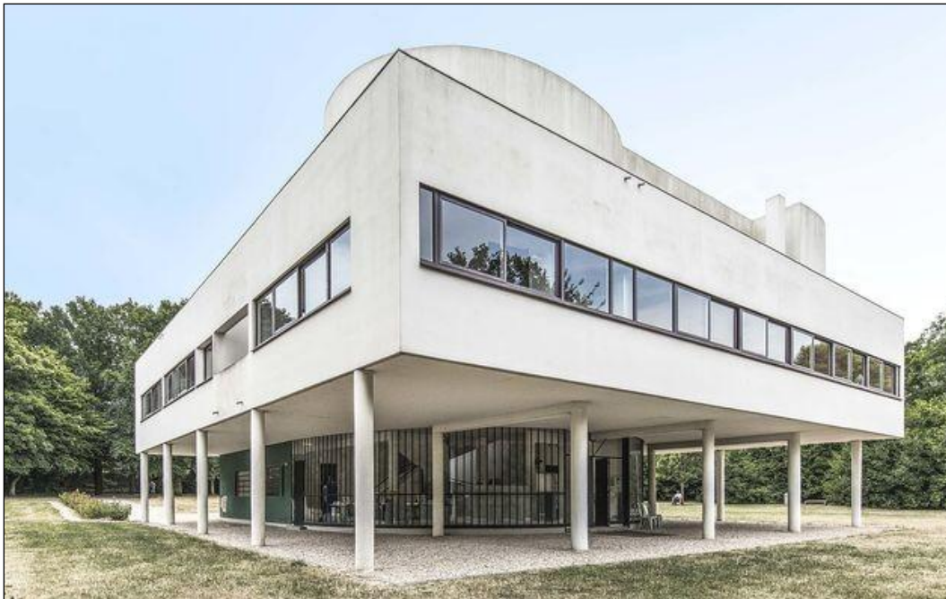
Plate 17 - Villa Savoye, 82 Rue de Villiers, 78300 Poissy, France, Le Corbusier, architect, built 1928-1931. (Reproduced from https://www.phaidon.com/agenda/architecture/articles/2019/february/04/le-corbusiers-grand-designs-villa-savoye/ .)
