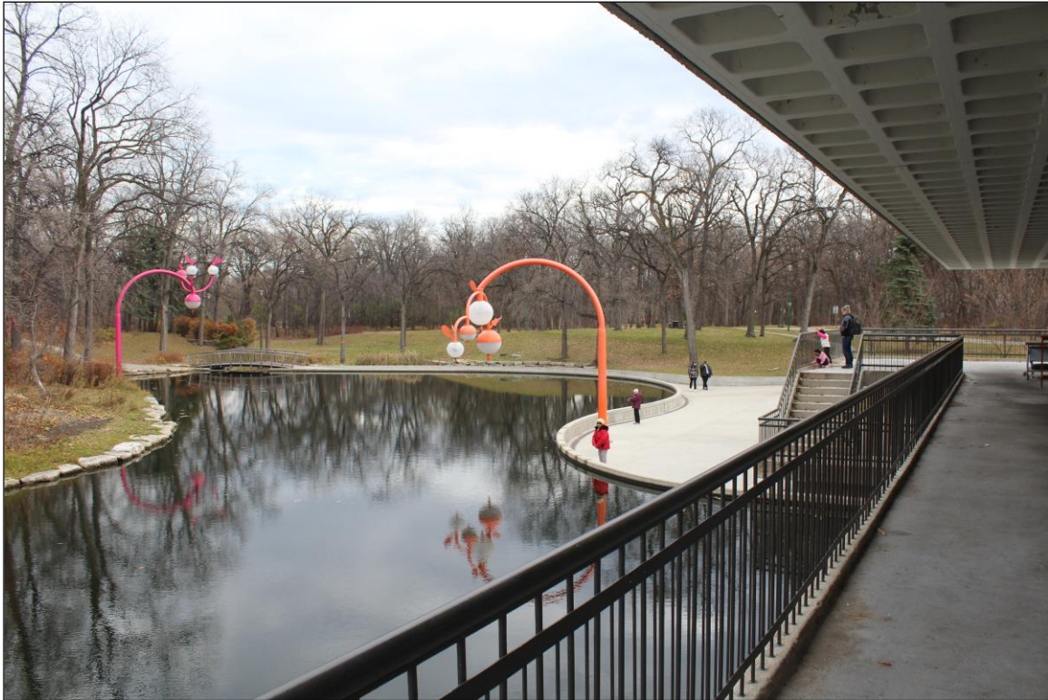
Plate 28 – Peguis Pavilion, Kildonan Park, 2015 Main Street, looking east from the deck, 2022. ( M. Peterson, 2022. )
