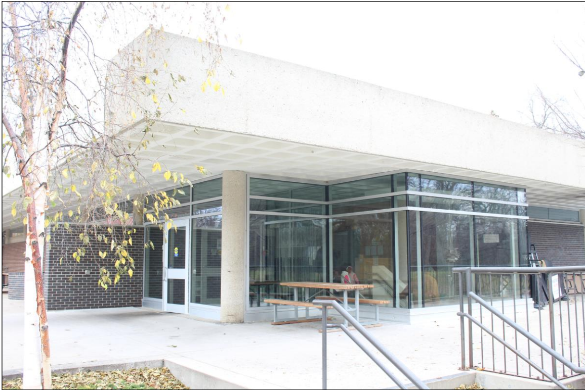
Plate 30 – Peguis Pavilion, Kildonan Park, 2015 Main Street, southeast corner entrance, 2022. ( M. Peterson, 2022. )
