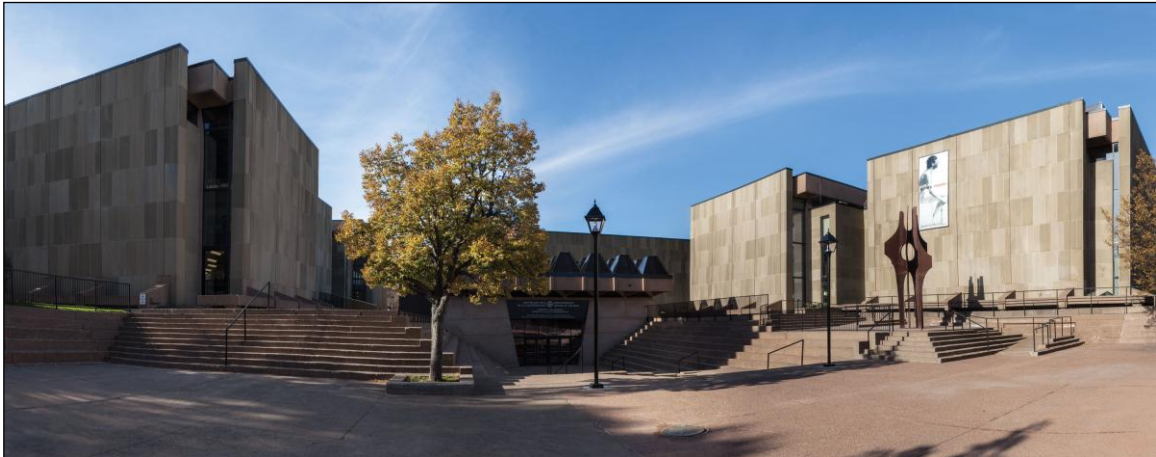
Plate 16 – Confederation Centre of the Arts, Charlottetown, P.E.I., opened in 1964, designated a National Historic Site in 2003 because, according to the Historic Sites and Monuments Board of Canada, “it is a distinguished example of Brutalist architecture in Canada.” (Photograph by Centre des arts de la Confédération, World Architecture website, no date.)
