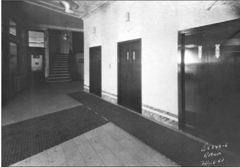
Plate 27 – Confederation Life Building, 457 Main Street, main floor, updated elevator lobby, 1940. (City of Winnipeg.)
