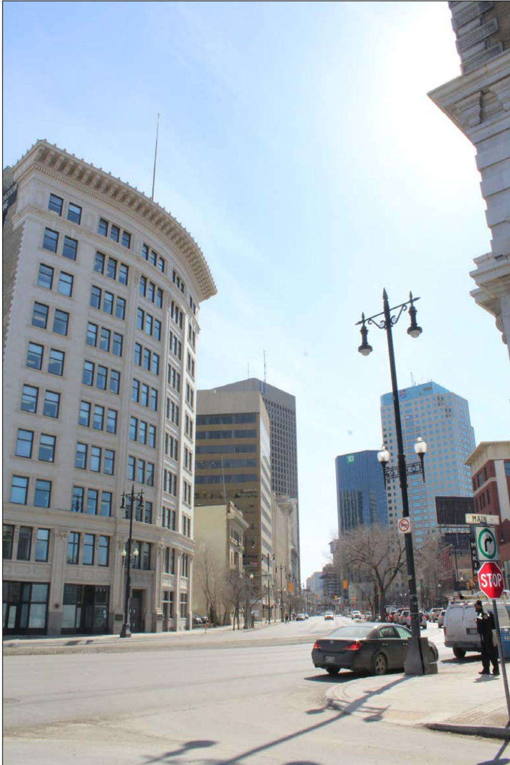
Plate 30 – Main Street, looking south from William Avenue, 2020. (M. Peterson, 2020.)
