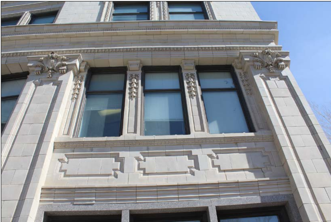
Plate 16 – Confederation Life Building, 457 Main Street, front (west) façade, terra cotta detail, 2020. (M. Peterson, 2020.)
