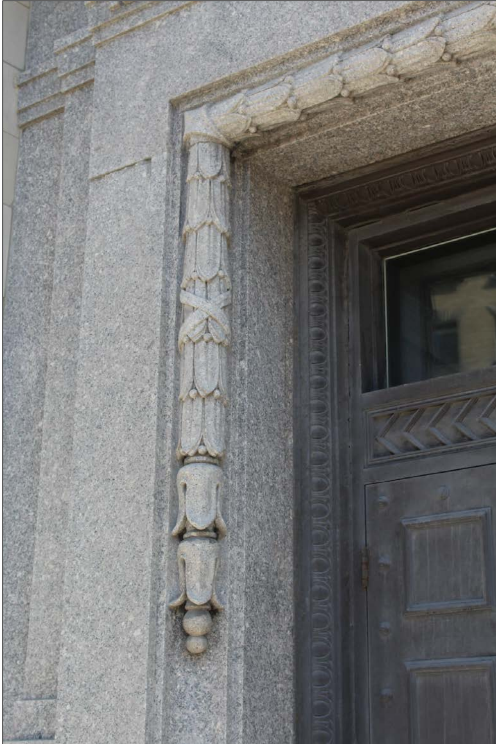
Plate 17 – Confederation Life Building, 457 Main Street, front (west) façade ground floor entrance detail, 2020. (M. Peterson, 2020.)
