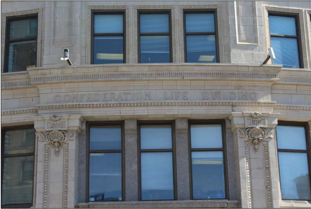
Plate 18 – Confederation Life Building, 457 Main Street, front (west) façade, main entrance detail, 2020. (M. Peterson, 2020.)
