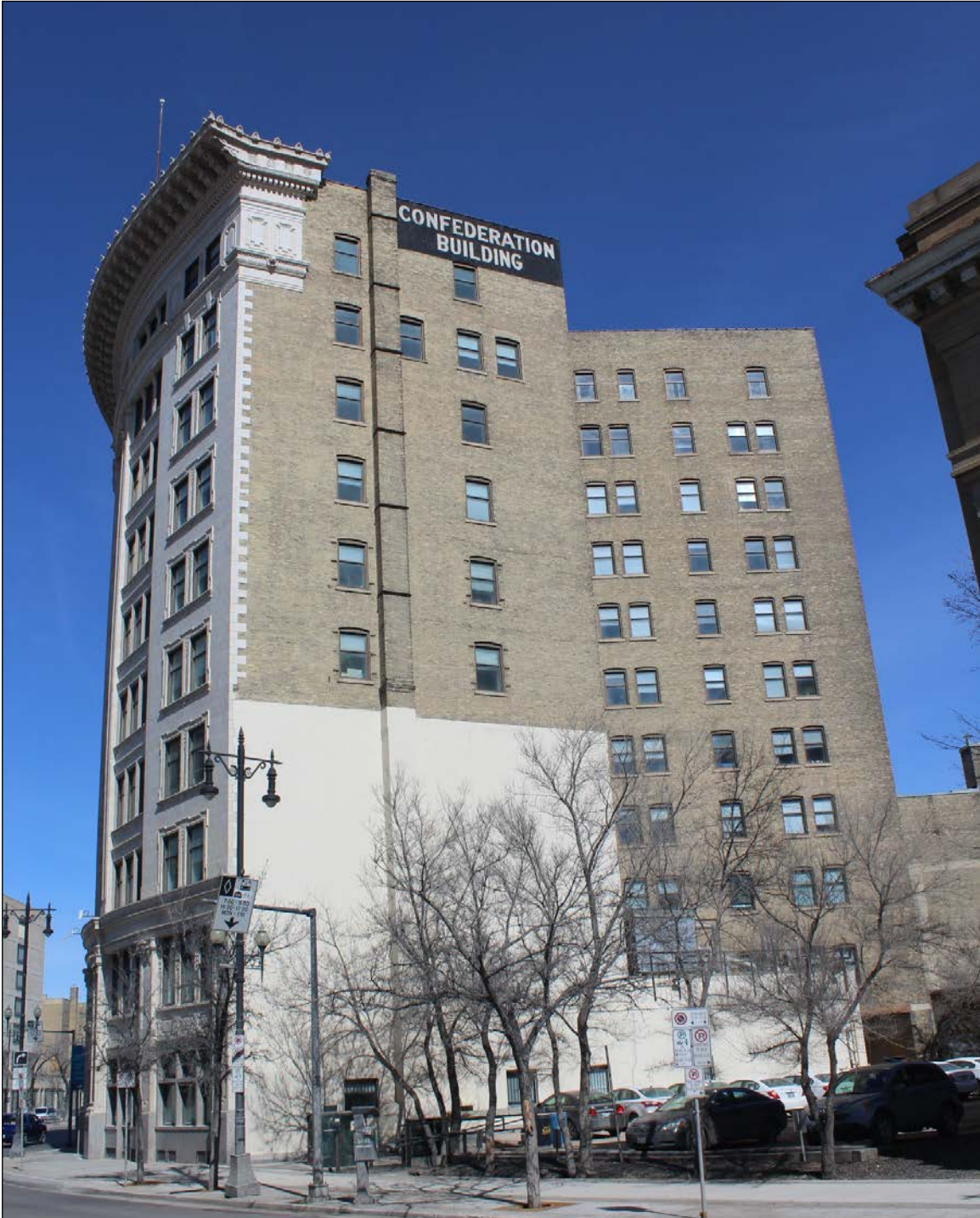
Plate 22 – Confederation Life Building, 457 Main Street, south façade, 2020. ( M. Peterson, 2020. )
