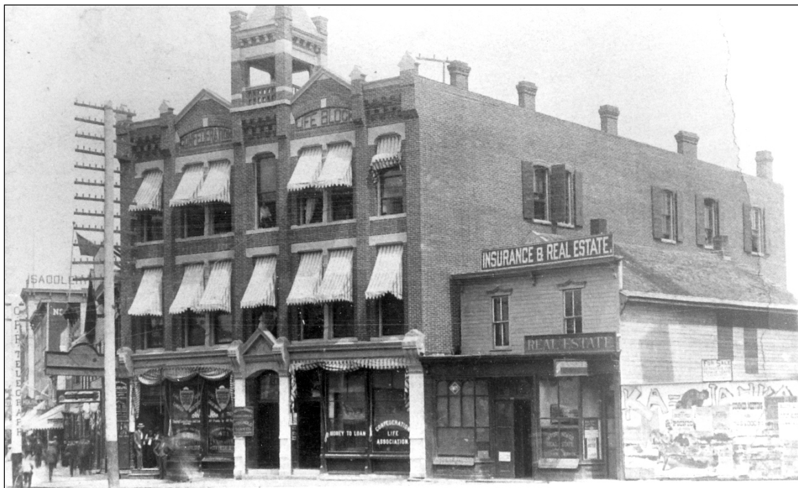
Plate 36 – Confederation Life Block, 471 Main Street, ca.1900. ( City of Winnipeg. )
