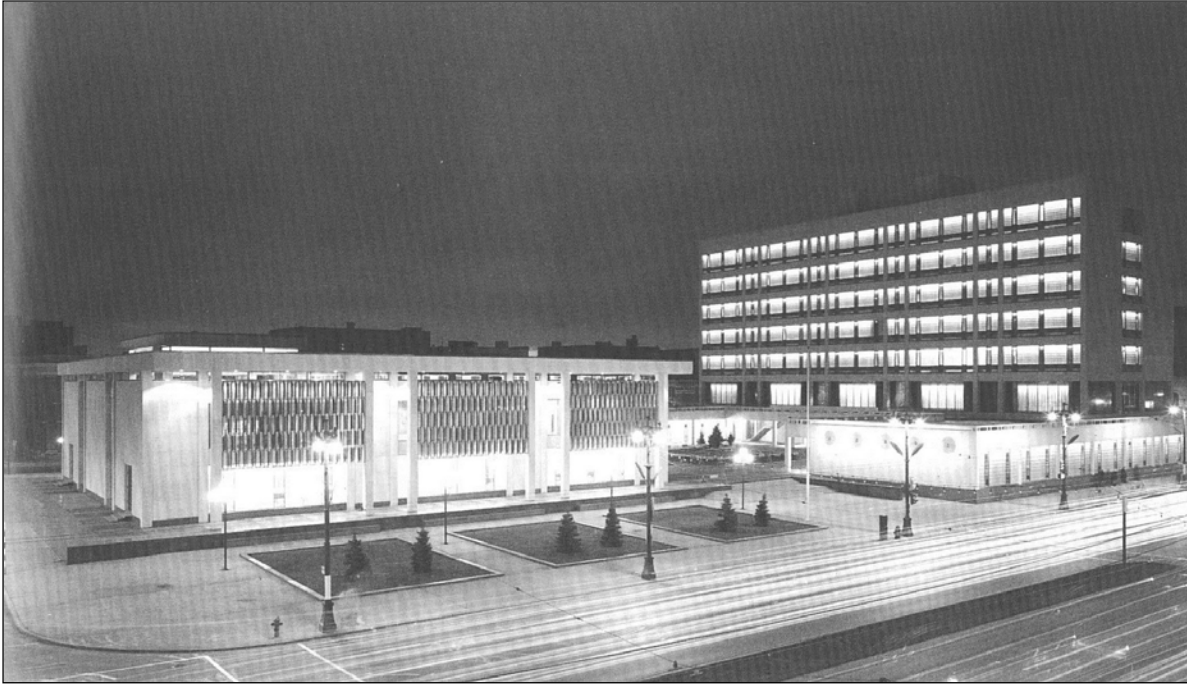
Plate 17 – City Hall, shortly after completion in 1964. (Photograph by Henry Kalen, 460L2.1-12, reproduced from Serena Keshavjee (ed.), Winnipeg Modern: Architecture 1945-1975 [Winnipeg, MB: University of Manitoba Press, 2006], p. 47.)
