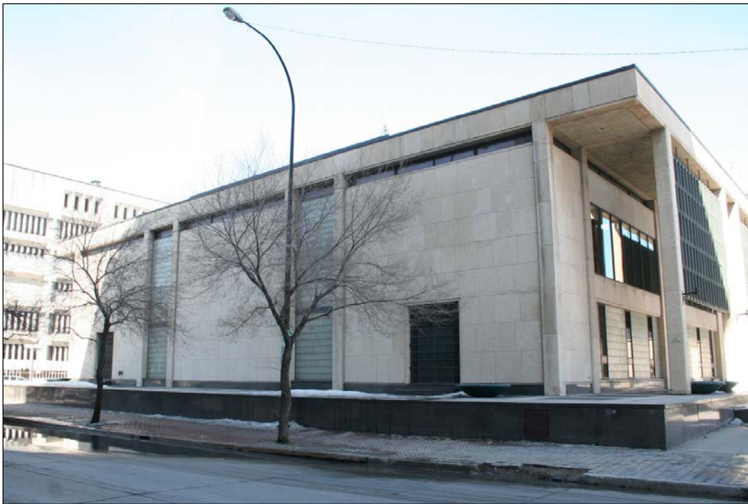
Plate 20 – City Hall, Council Building, 510 Main Street, south façade, 2014. (M. Peterson, 2014.)
