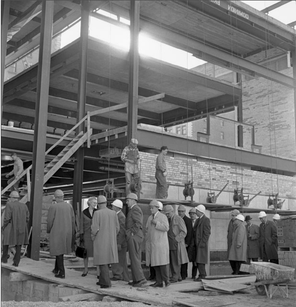
Plate 16 – Mayor Juba and Winnipeg City Councillors touring the City Hall construction site, June 11, 1963. ( Reproduced from the Winnipeg Tribune Collection, University of Manitoba Archives, PC 18-1587-001. )
