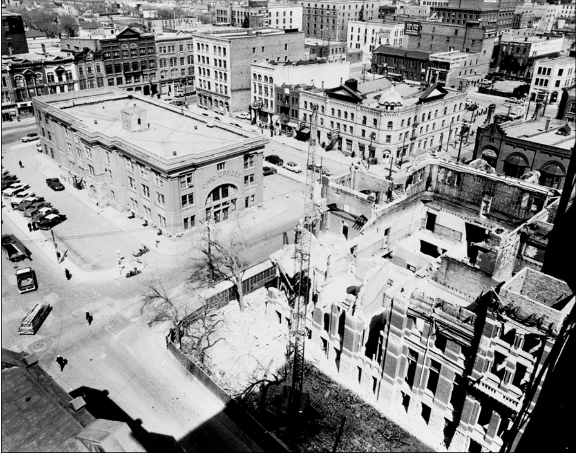
Plate 12 – Civic Office Building, Princess Street, during the 1962 demolition of the “Gingerbread” City Hall. ( City of Winnipeg. )
