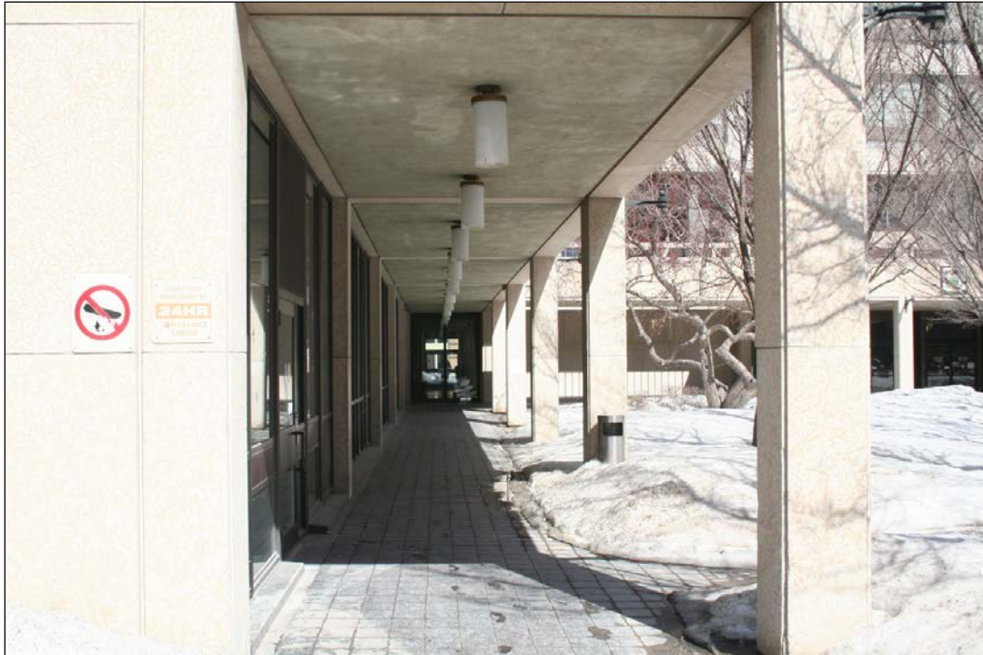
Plate 29 – City Hall, Administration Building, 510 Main Street, north façade, 2014. ( M. Peterson, 2014. )
