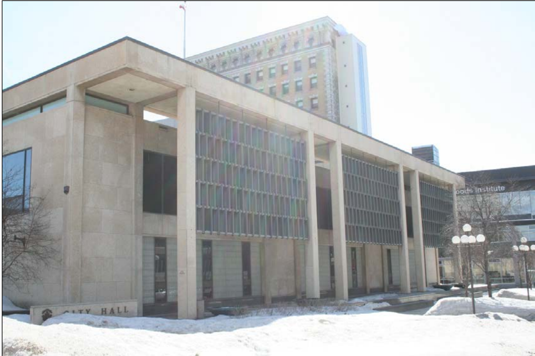
Plate 19 – City Hall, Council Building, 510 Main Street, north side, 2014. (M. Peterson, 2014.)
