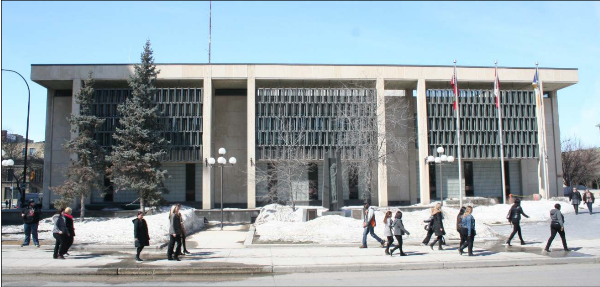
Plate 21 – City Hall, Council Building, 510 Main Street, east façade, 2014. (M. Peterson, 2014.)
