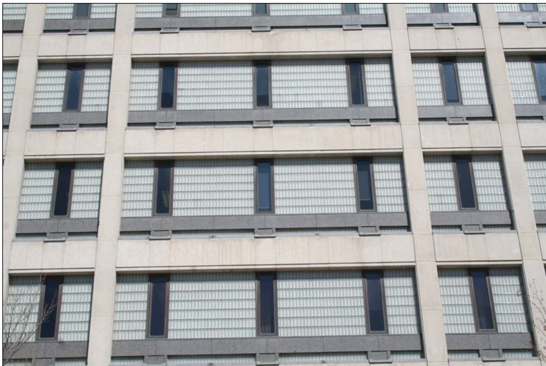
Plate 26 – City Hall, Administration Building, 510 Main Street, detail of south façade, 2014. ( M. Peterson, 2014. )
