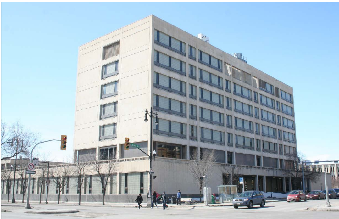
Plate 28 – City Hall, Administration Building, 510 Main Street, north and west façades, 2014. ( M. Peterson, 2014. )
