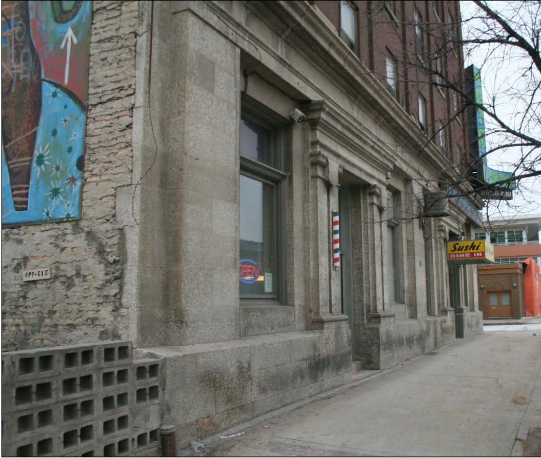
Plate 11 – McLaren Hotel, 554 Main Street, detail of east façade, 2014. (M. Peterson, 2014.)
