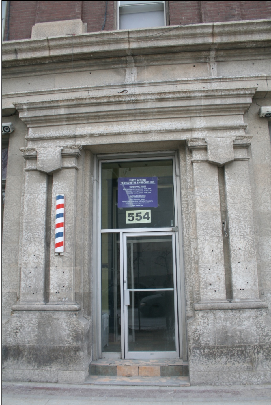
Plate 12 – McLaren Hotel, 554 Main Street, south door, east façade, 2014. (M. Peterson, 2014.)
