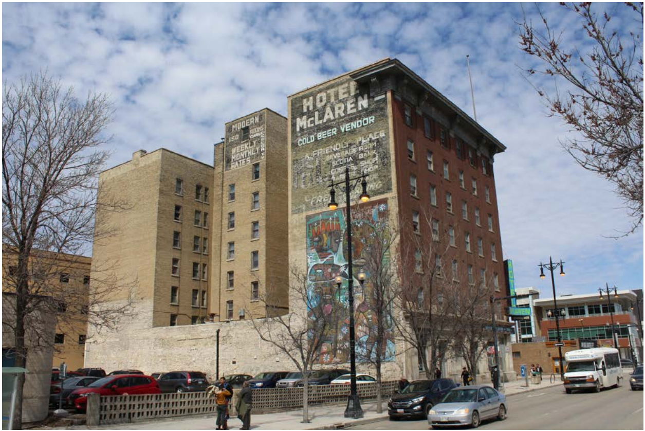
Plate 16 – McLaren Hotel, 554 Main Street, east and south façades, 2019. ( M. Peterson, 2019. )
