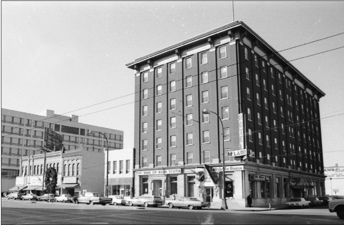
Plate 28 – McLaren Hotel, 554 Main Street, ca.1967, with the Bank of Nova Scotia and Salisbury House Restaurant occupying the ground floor commercial space. ( City of Winnipeg. )
