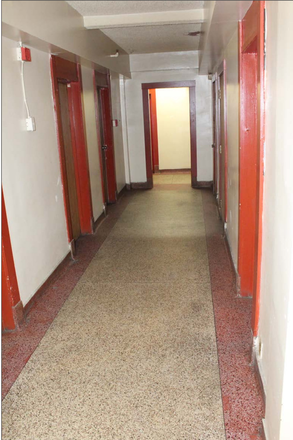
Plate 22 – McLaren Hotel, 554 Main Street, second floor hallway with terrazzo flooring, 2019. (M. Peterson, 2019.)
