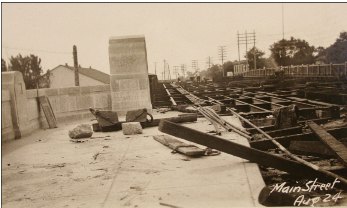
Plate 11 – Construction of the Main Street Bridge, August 24, 1931 with stone pylon/solid stone wall element in the foreground. ( Archives of Manitoba, “Winnipeg-Bridges-Main 2-Construction 1932-#35.” )
