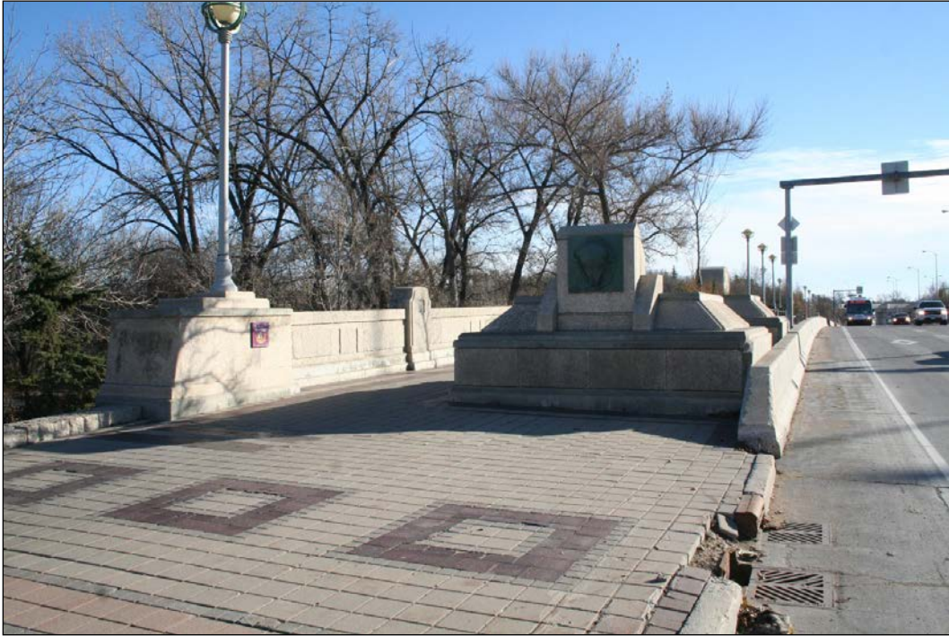
Plate 16 – Northeast corner, Queen Elizabeth Way, 2013, showing 1930s era solid, low stone wall. (M. Peterson, 2013.)
