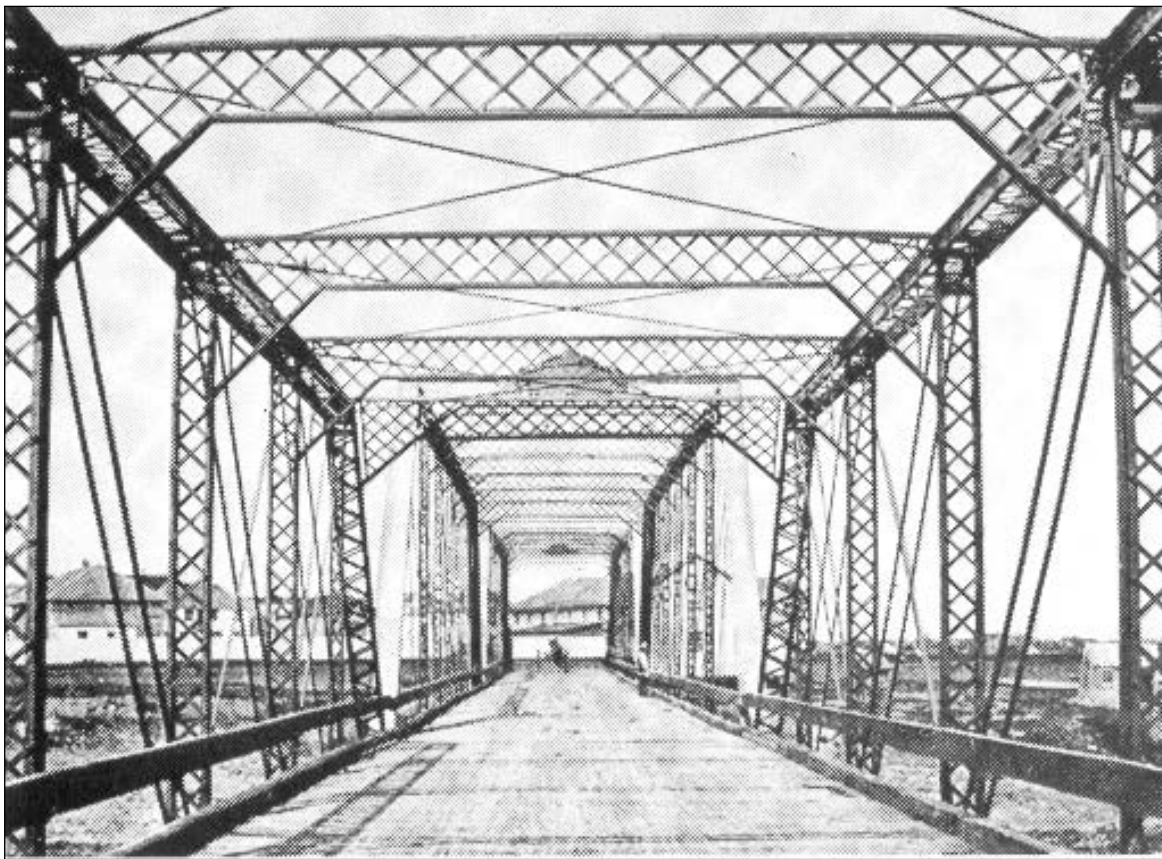
Plate 1 – The first Assiniboine (Main Street) Bridge, with Upper Fort Garry in the background, n.d. (Reproduced from Winnipeg 100 [Winnipeg: Winnipeg Free Press, 1973], p. 10.)
