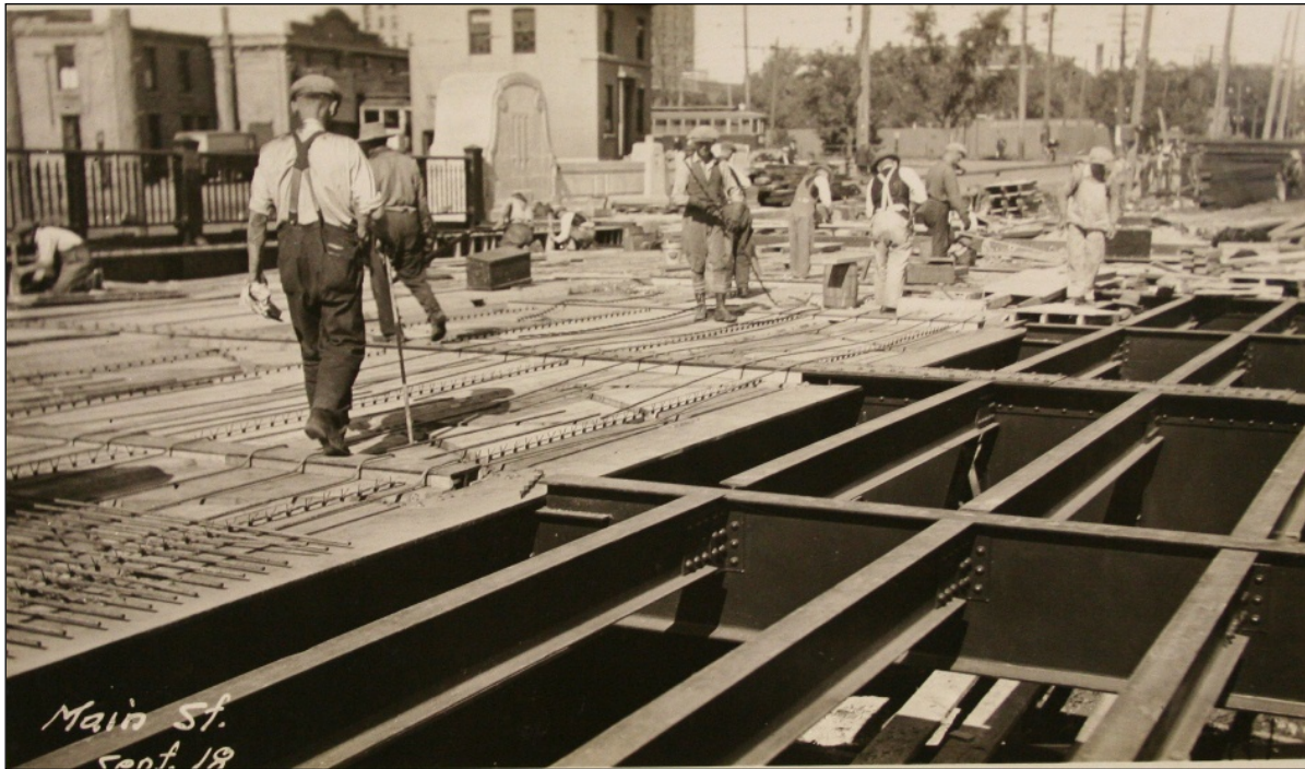
Plate 12 – Construction of the Main Street Bridge, September 18, 1931 with metal railing and stone elements in the background. ( Archives of Manitoba, “Winnipeg-Bridges-Main 2-Construction 1932-#37.” )
