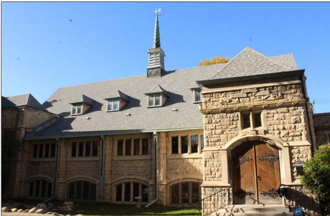
Plate 11 – St. Luke’s Anglican Church, 130 Nassau Street North, southeast entrance of the 1914 addition, 2017. (M. Peterson, 2017.)
