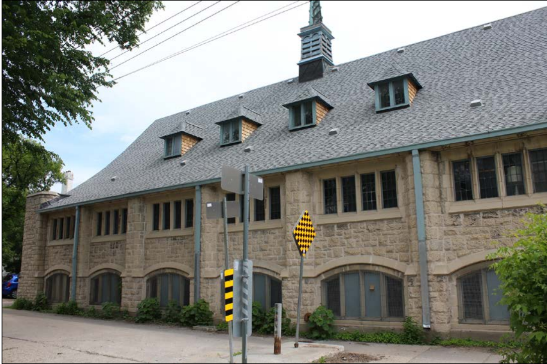
Plate 10 – St. Luke’s Anglican Church, 130 Nassau Street North, north façade of 1914 addition, 2016. (M. Peterson, 2016.)
