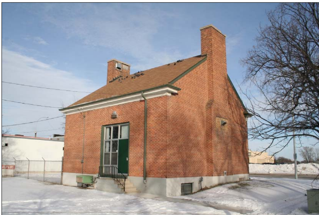
Plate 15 – Former Winnipeg Electric Company Osborne Street Substation, 265 Osborne Street, rear (west) and south façades, 2012. (M. Peterson, 2012.)
