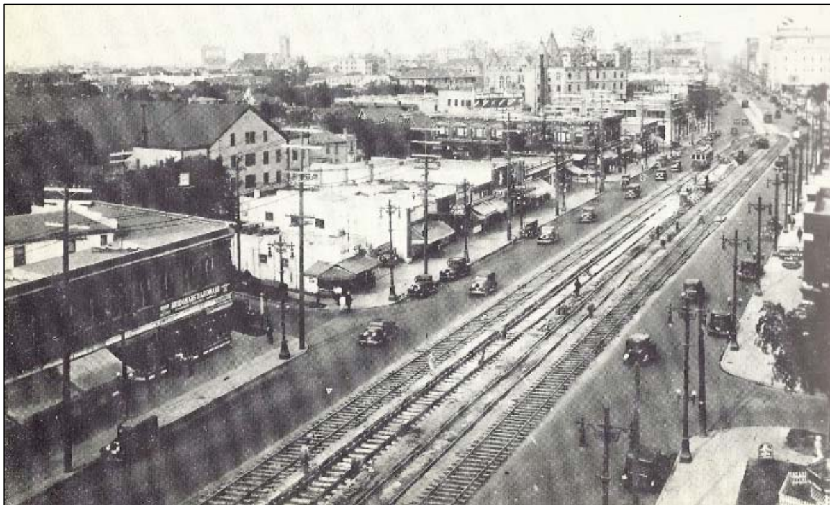
Plate 7 – Portage Avenue, looking east from Sherbrook Street in August 1930. The middle sets of tracks are being repaired/replaced, while the streetcars run on temporary tracks laid beside on the pavement. ( Foote Collection No. 1506, Archives of Manitoba. )
