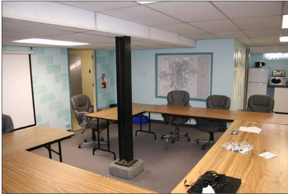
Plate 20 – Former Winnipeg Electric Company Osborne Street Substation, 265 Osborne Street, basement, 2012. (M. Peterson, 2012.)
