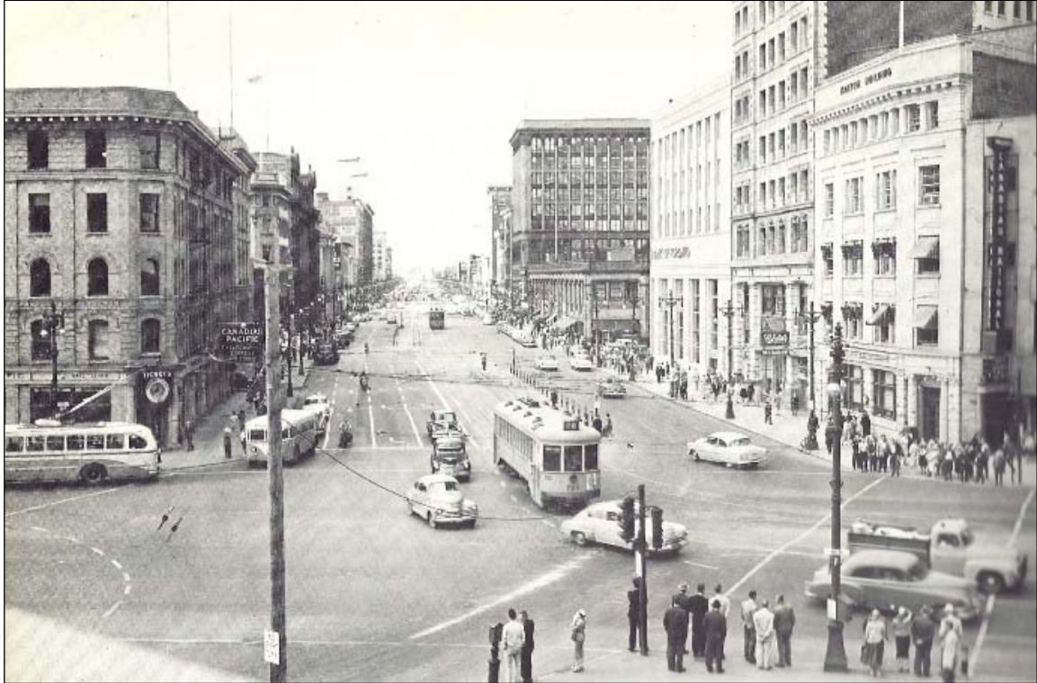
Plate 8 – This ca.1950 image of Portage and Main shows a number of interesting items: trolley coaches turning south onto Main Street, a streetcar turning north onto Main Street and behind it, the median loading area for streetcar passengers. ( Winnipeg Transit System images, reproduced from J.E. Baker, Winnipeg's Electric Transit. The Story of Winnipeg's Streetcars and Trolley Busses [West Hill, On: Railfare Enterprises, 1982], p. 102. )
