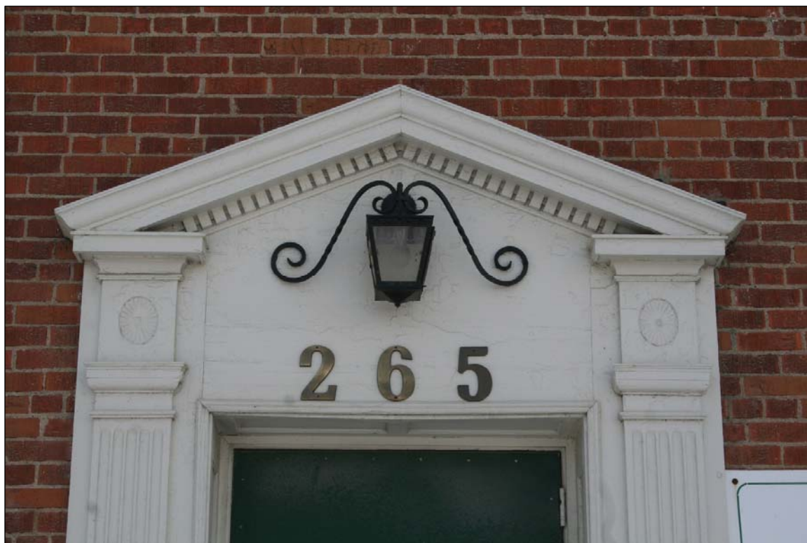
Plate 13 – Former Winnipeg Electric Company Osborne Street Substation, 265 Osborne Street, front entrance detail, 2012. (M. Peterson, 2012.)
