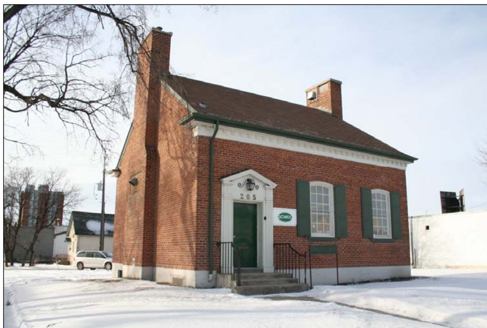
Plate 12 – Former Winnipeg Electric Company Osborne Street Substation, 265 Osborne Street, front (east) and south façades, 2012. (M. Peterson, 2012.)
