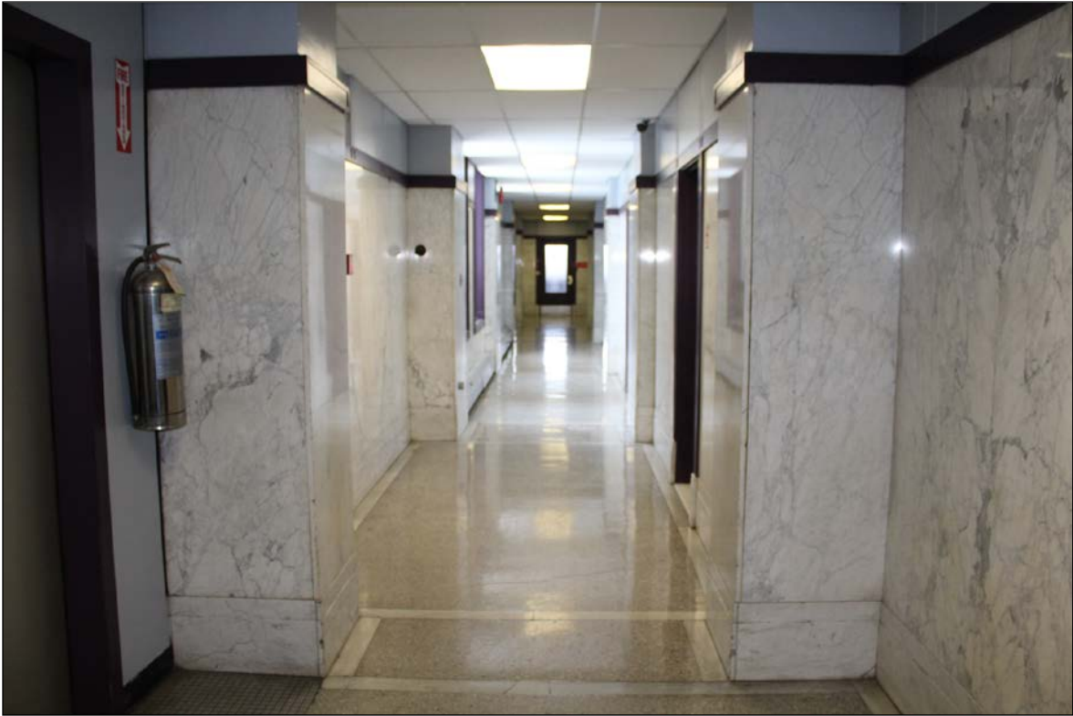
Plate 22 – Sterling Bank Building, 283 Portage Avenue, third floor hallway, 2015. ( M. Peterson, 2015. )
