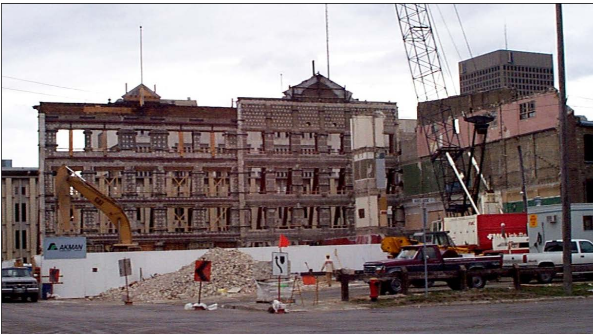
Plate 18– Princess Street Block, spring 2001 stabilization and demolition. (M. Peterson, 2001.)
