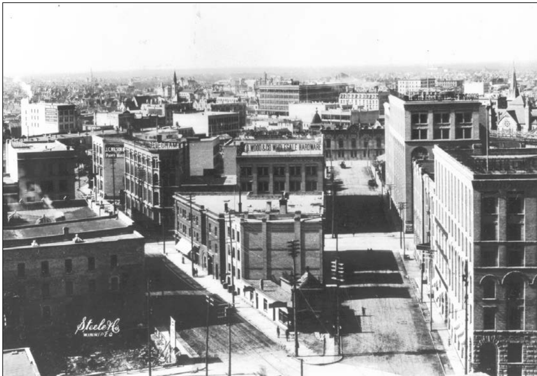
Plate 2 – Warehouse District, ca.1905, showing the scale of development over the previous 20 years. (Courtesy of the Archives of Manitoba.)
