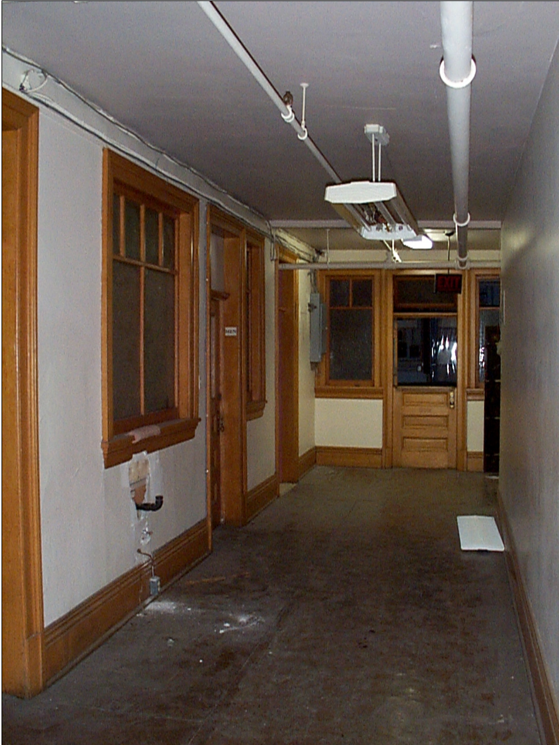
Plate 15 – Exchange Building, 160 Princess Street, second floor hallway, 1998. ( M. Peterson, 1998. )
