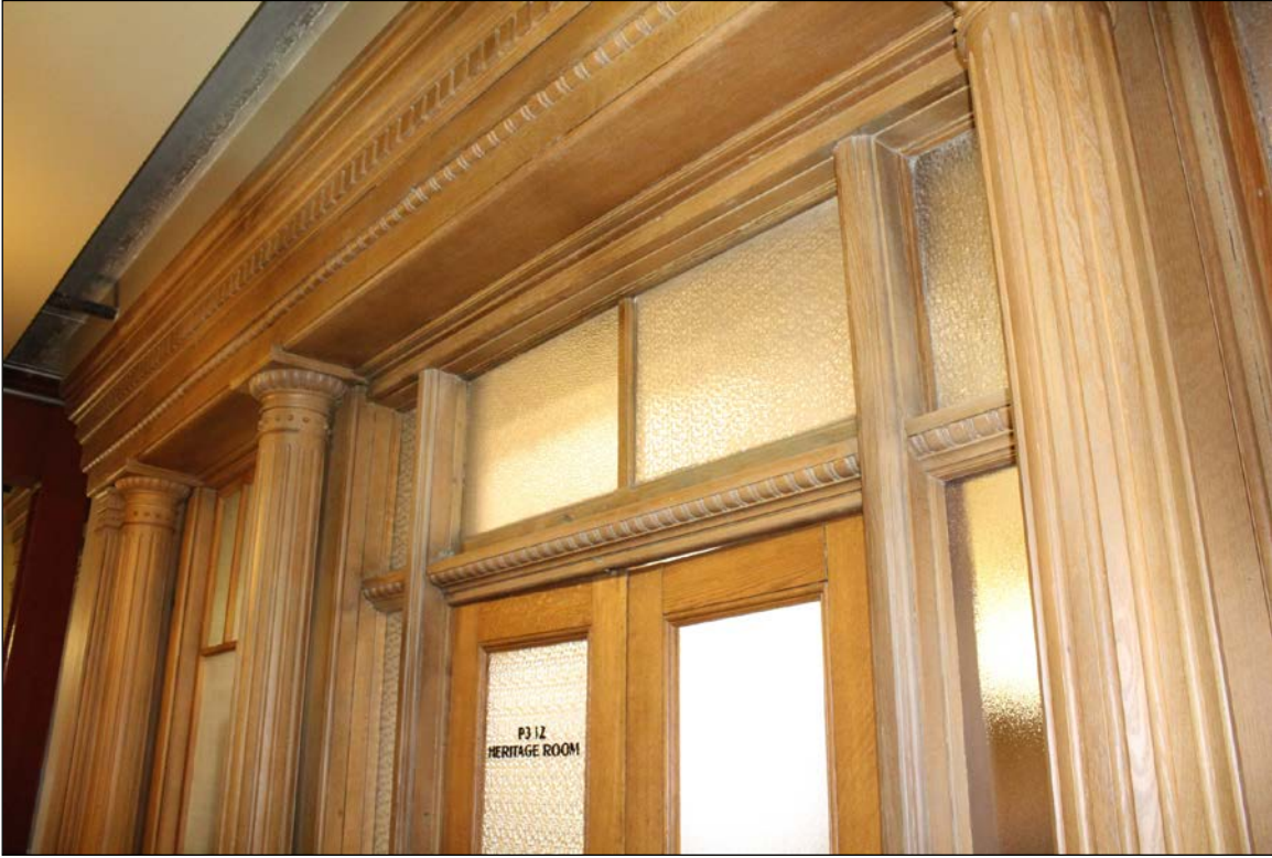
Plate 27 – Red River College Princess Street Campus, 140 Princess Street, original 160 Princess Street third floor oak detailing rebuilt in its original location, 2019. (M. Peterson, 2019.)
