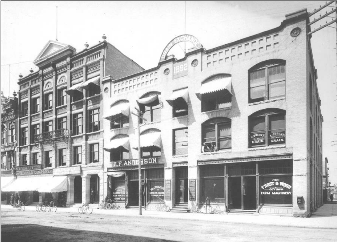
Plate 6 – Original Grain Exchange Building, 164 Princess Street (right) and annex, 160 Princess Street (left), ca.1900. A fourth storey was added to 164 Princess Street in 1902. (William H. Carre, Art Work on Winnipeg, Manitoba, Canada [Winnipeg, MB: William H. Carre Company, 1900], Part 5, p. 2.)
