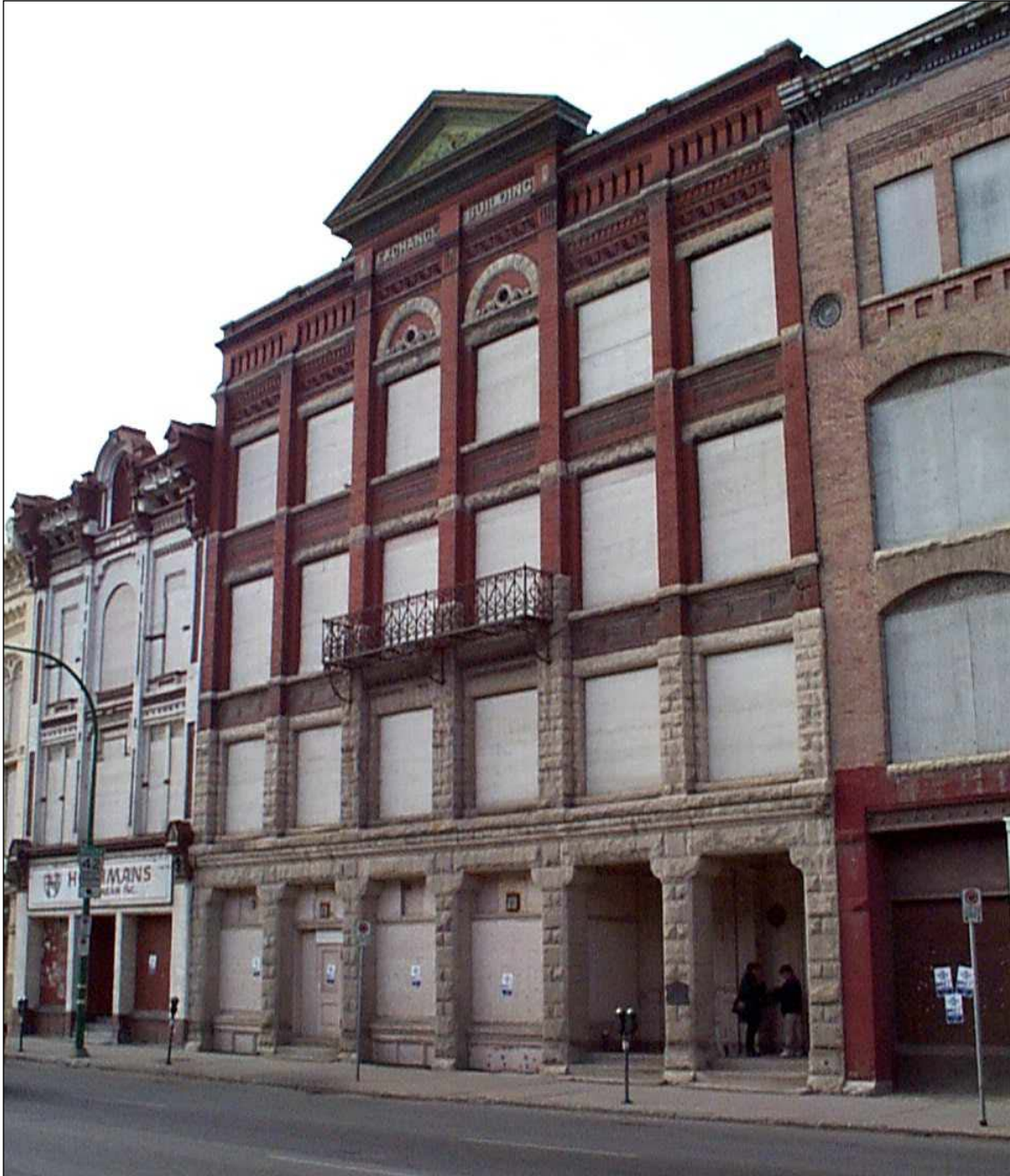
Plate 10 – Exchange Building, 160 Princess Street, front (east) façade, 2000. ( M. Peterson, 2000. )
