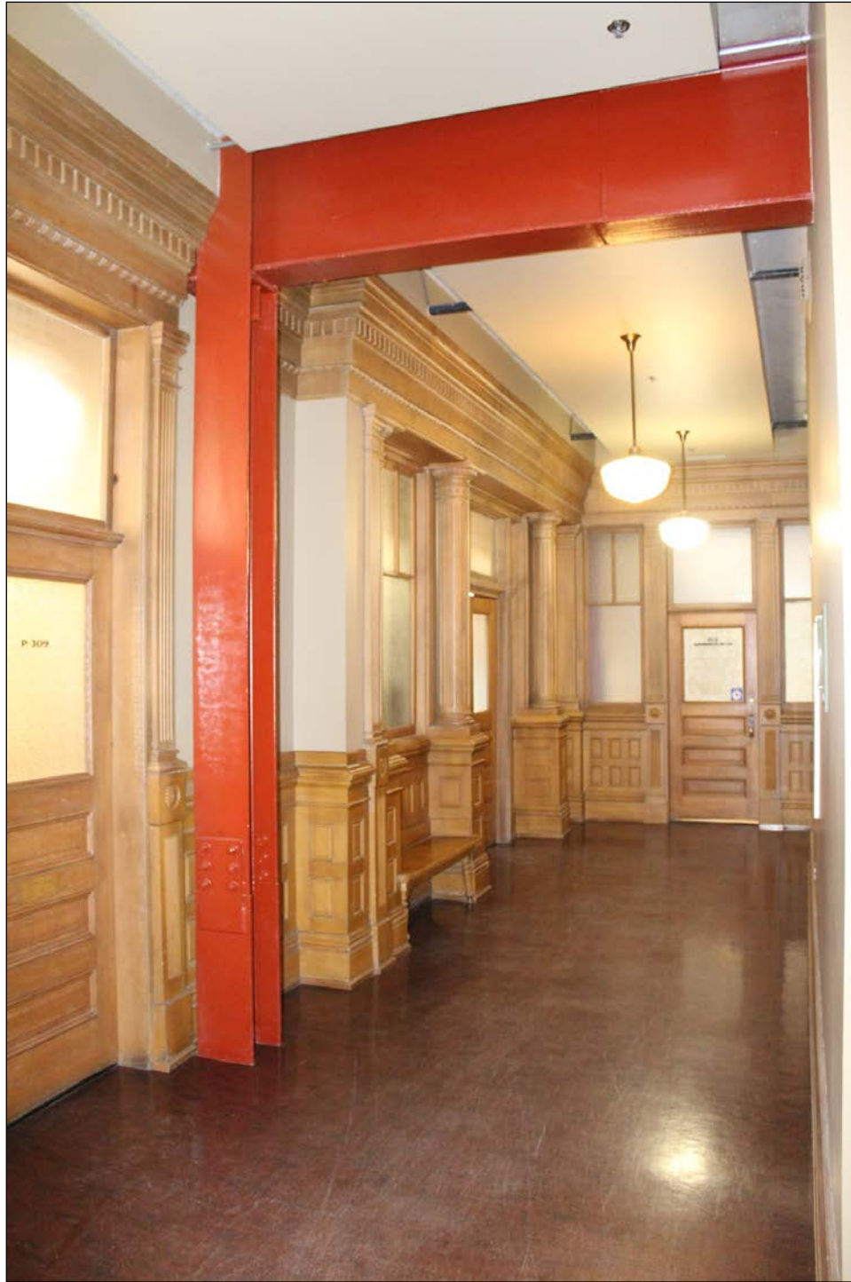
Plate 26 – Red River College Princess Street Campus, 140 Princess Street, original 160 Princess Street third floor oak detailed hallway rebuilt in its original location, 2019. ( M. Peterson, 2019. )
