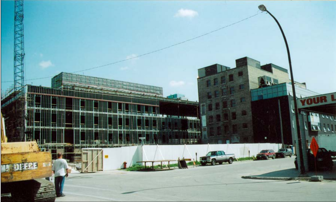
Plate 20 – Red River College Princess Street Campus, 140 Princess Street, construction of new building, rear (west) façade, 2001. ( M. Peterson, 2001. )
