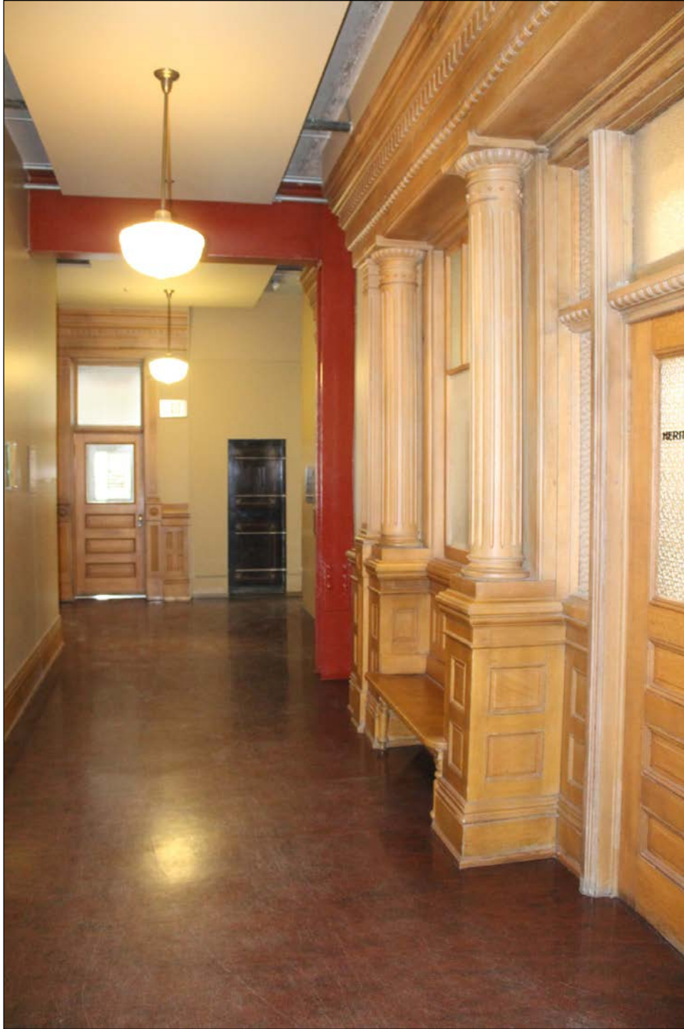
Plate 25 – Red River College Princess Street Campus, 140 Princess Street, original 160 Princess Street third floor oak detailed hallway rebuilt in its original location, 2019. ( M. Peterson, 2019. )
