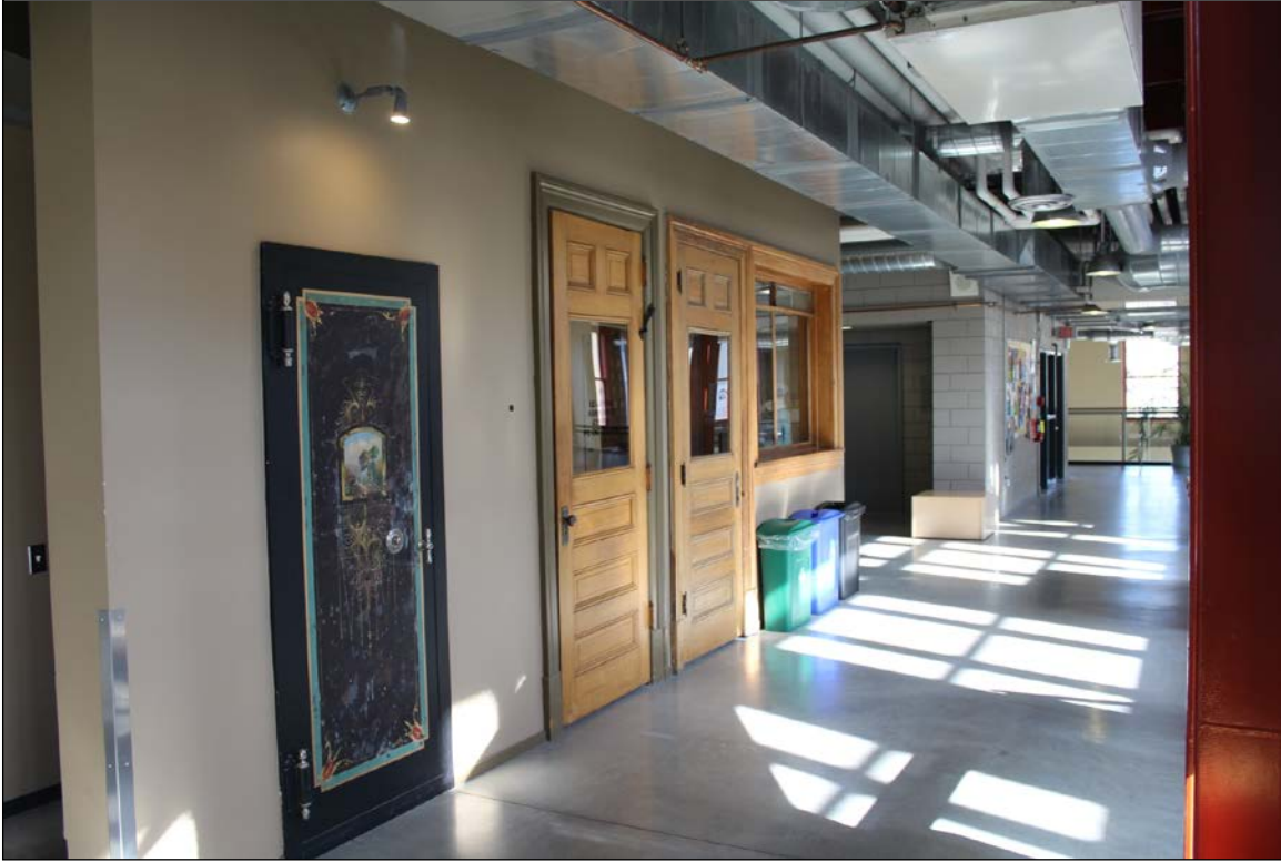
Plate 24 – Red River College Princess Street Campus, 140 Princess Street, second floor with original 160 Princess Street second floor vault doors and oak doors and trim reused, 2019. ( M. Peterson, 2019. )
