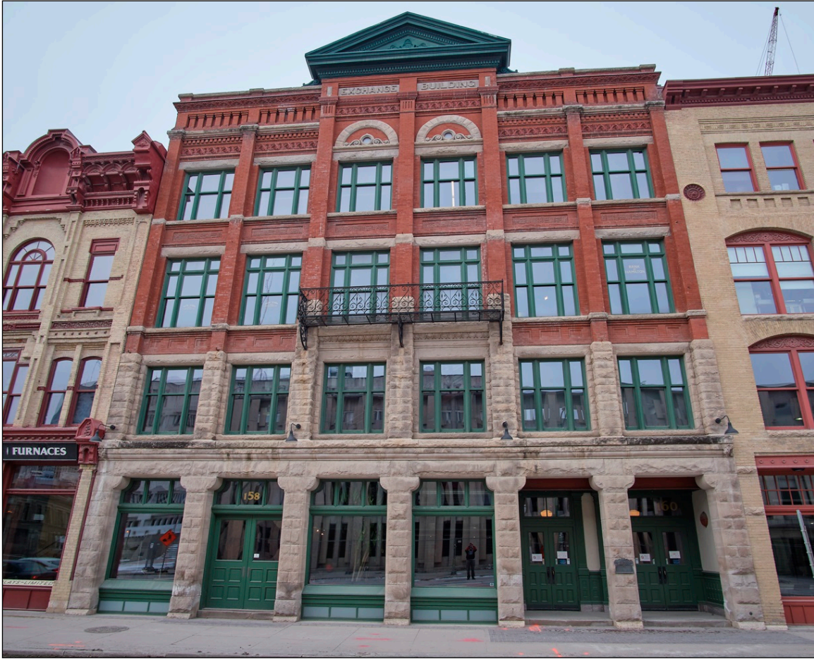
Plate 11 – Exchange Building, 160 Princess Street, front (east) façade, 2019. (G. Cline, 2019.)
