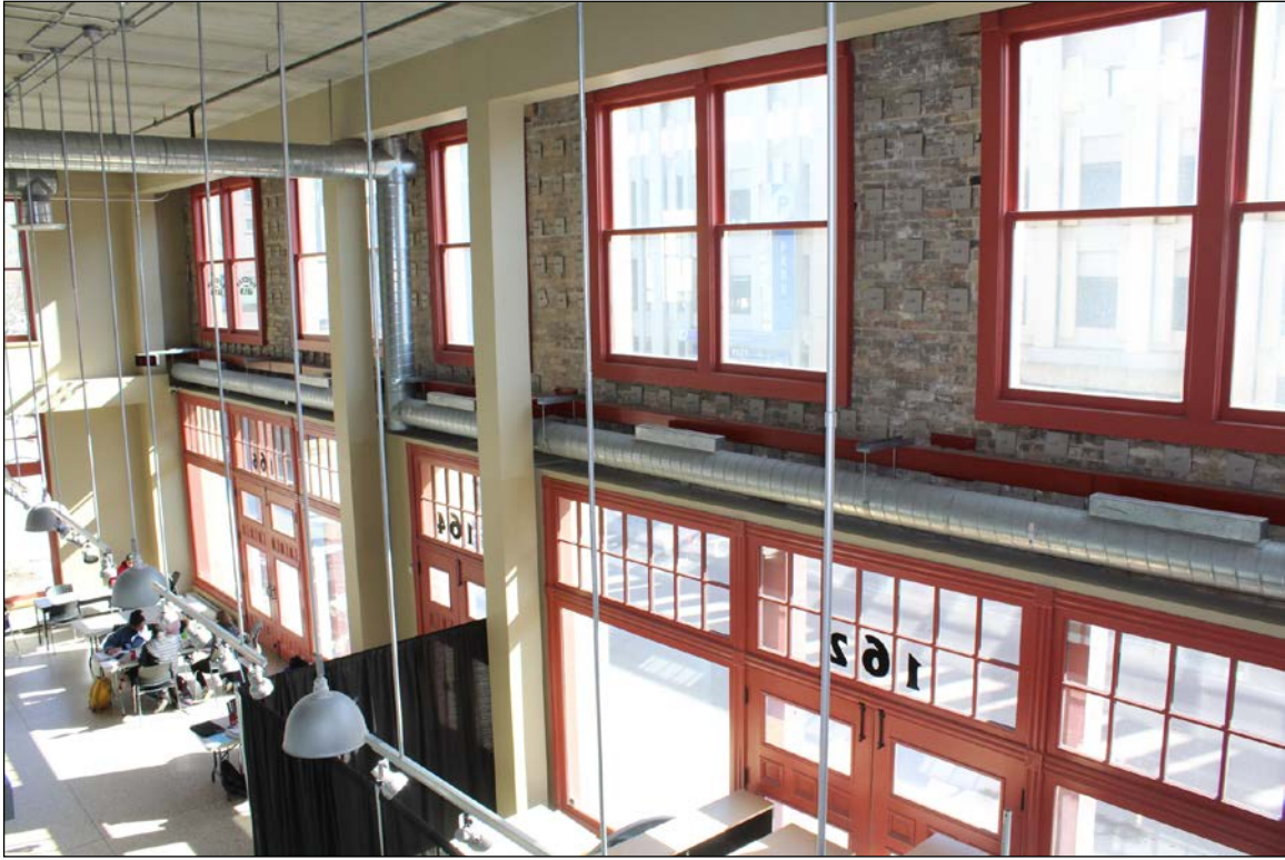
Plate 24 – Red River College Princess Street Campus, 140 Princess Street, main floor, 162-164 Princess Street, 2019. (M. Peterson, 2019.)
