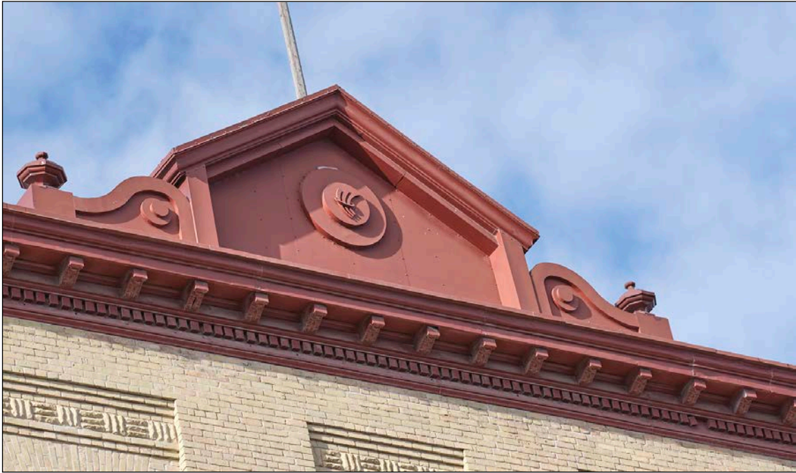
Plate 15 – Utility Building, 164 Princess Street, detail of rebuilt front (east) façade pediment with Red River College logo, 2019. ( G. Cline, 2019. )
