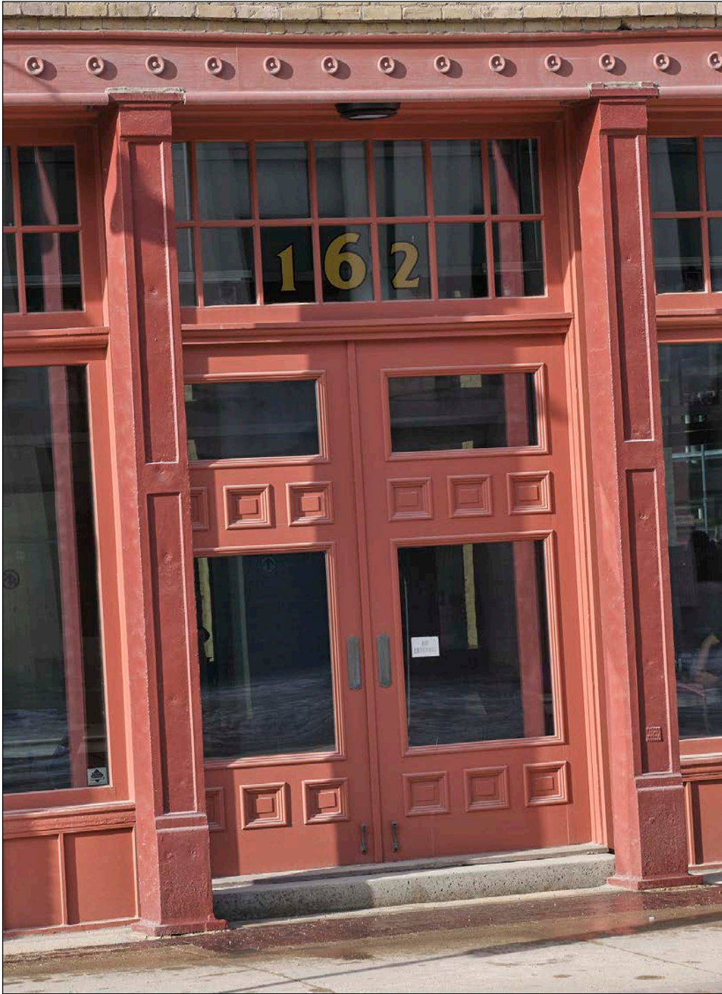
Plate 18 – Utility Building, 164 Princess Street, front (east) façade entrance, 2019. ( M. Peterson, 2019. )
