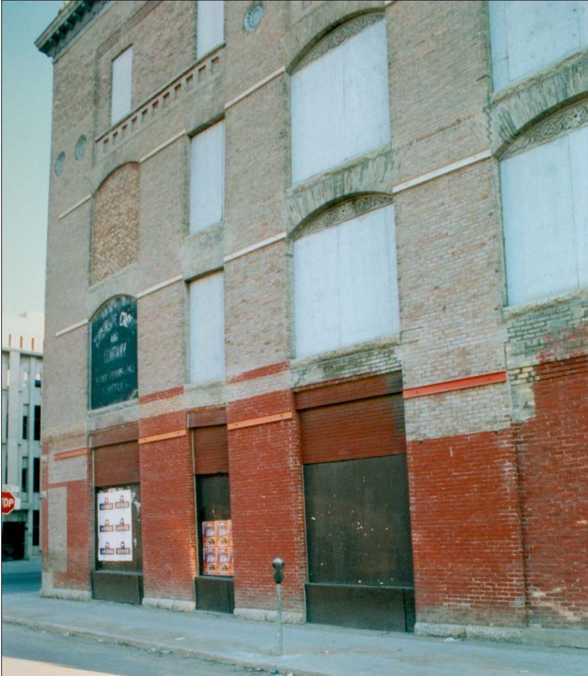
Plate 10 – Utility Building, 164 Princess Street, east end of the north façade, 1999. ( Eschmade, 1999, Image #77. )
