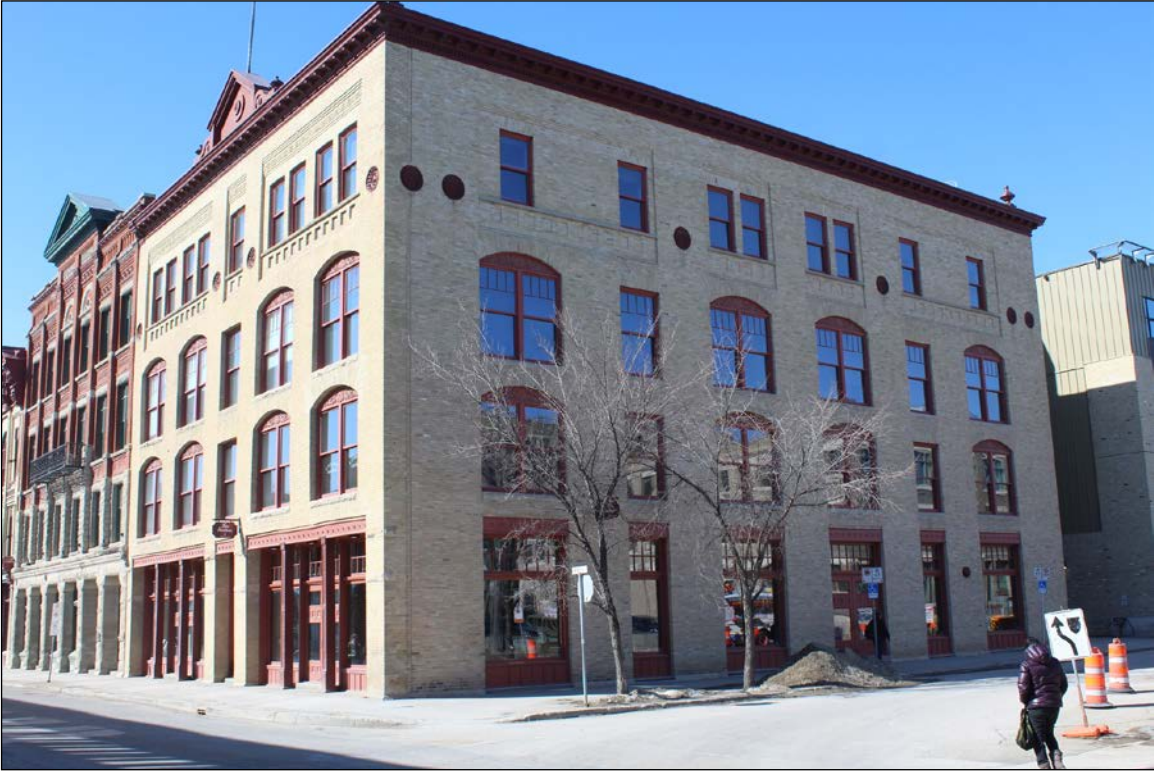
Plate 13 – Utility Building, 164 Princess Street, front (east) and north façades, 2019. ( M. Peterson, 2019. )
