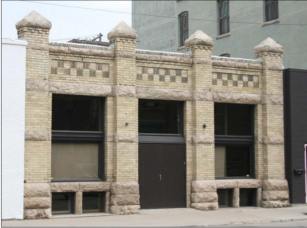
Plate 2 – Toronto Hide and Wool Company Building, 200 Princess Street, front (north) façade, 2014. (M. Peterson, 2014.)
