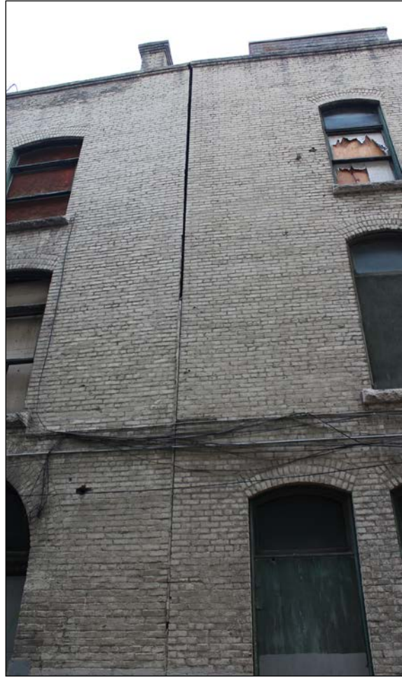
Plate 8 – McLaughlin Carriage Company Building, 208 Princess Street, cracks in the front (east) and rear (west) façades, 2015. ( M. Peterson, 2015. )
