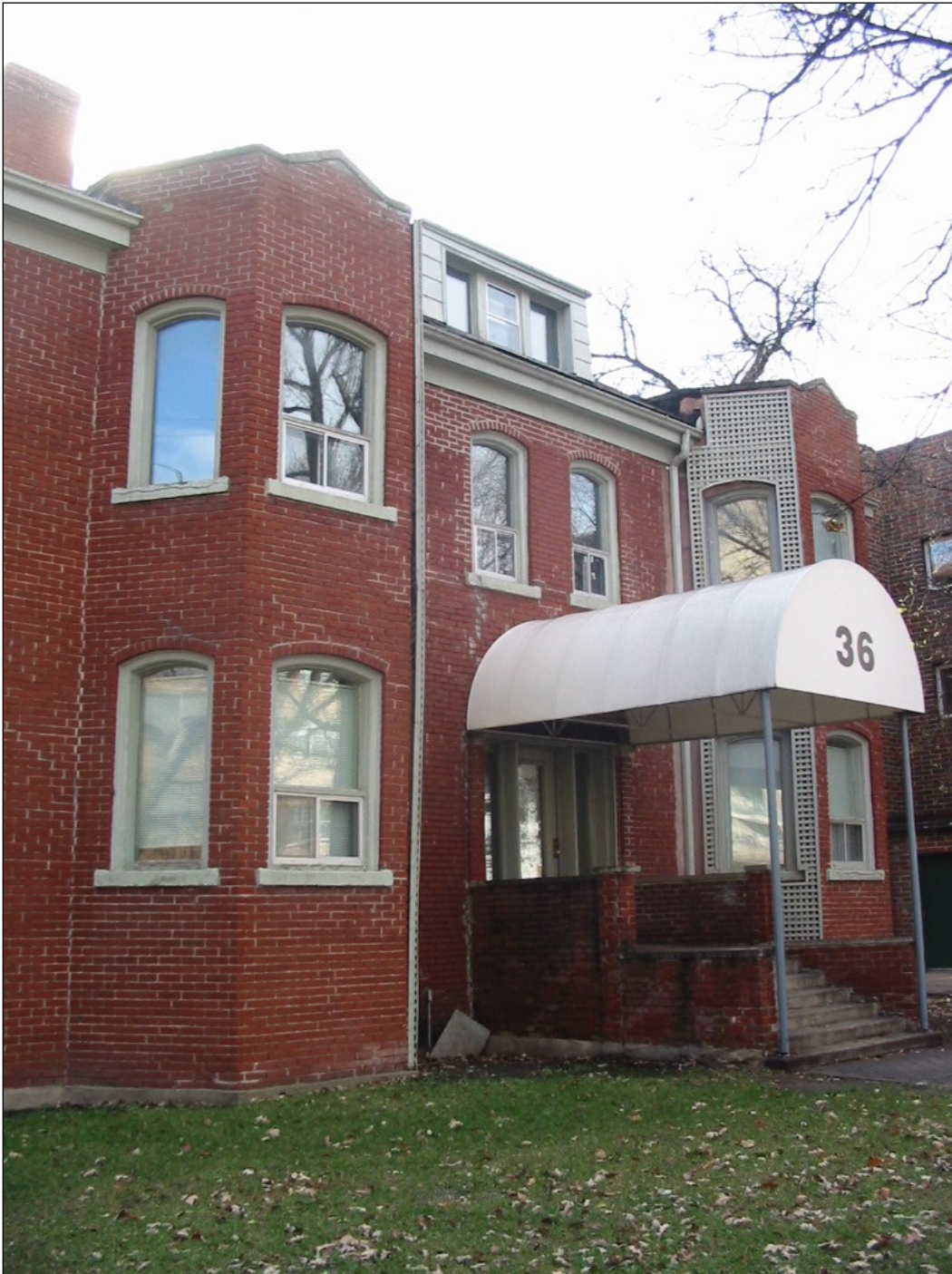
Plate 7 – John C. Falls House, 36 Roslyn Road, front (north) façade, 2004, showing the red brick, and bay window pediments. (M. Peterson, 2004.)
