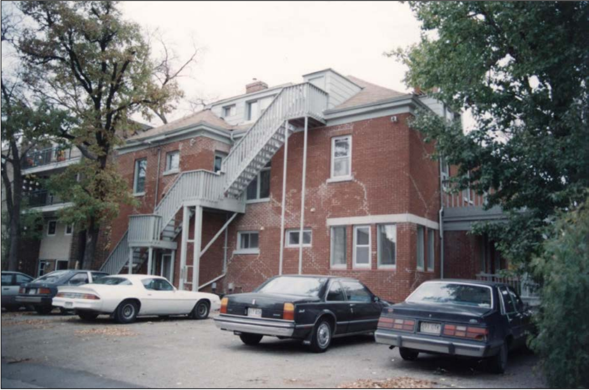
Plate 11 – John C. Falls House, 36 Roslyn Road, rear (south) façade, 1993. ( M. Peterson, 1993. )
