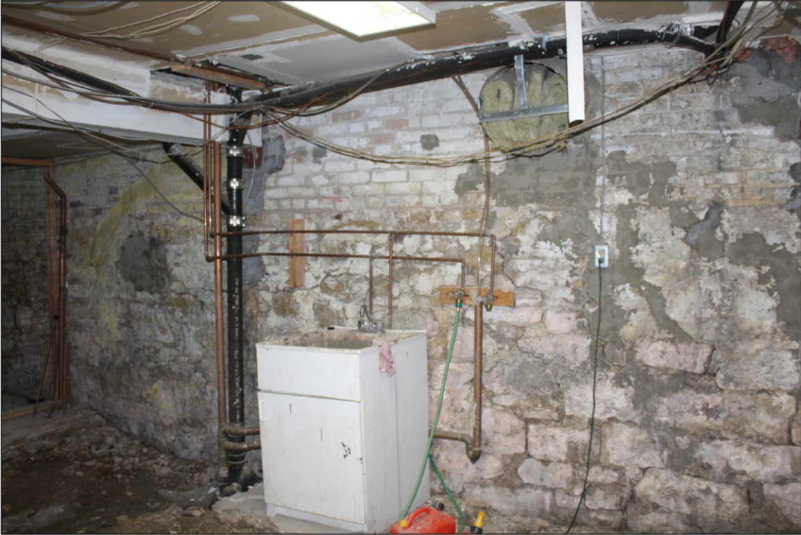
Plate 3 – John C. Falls House, 36 Roslyn Road, basement, 2021. (M. Peterson, 2021.)
