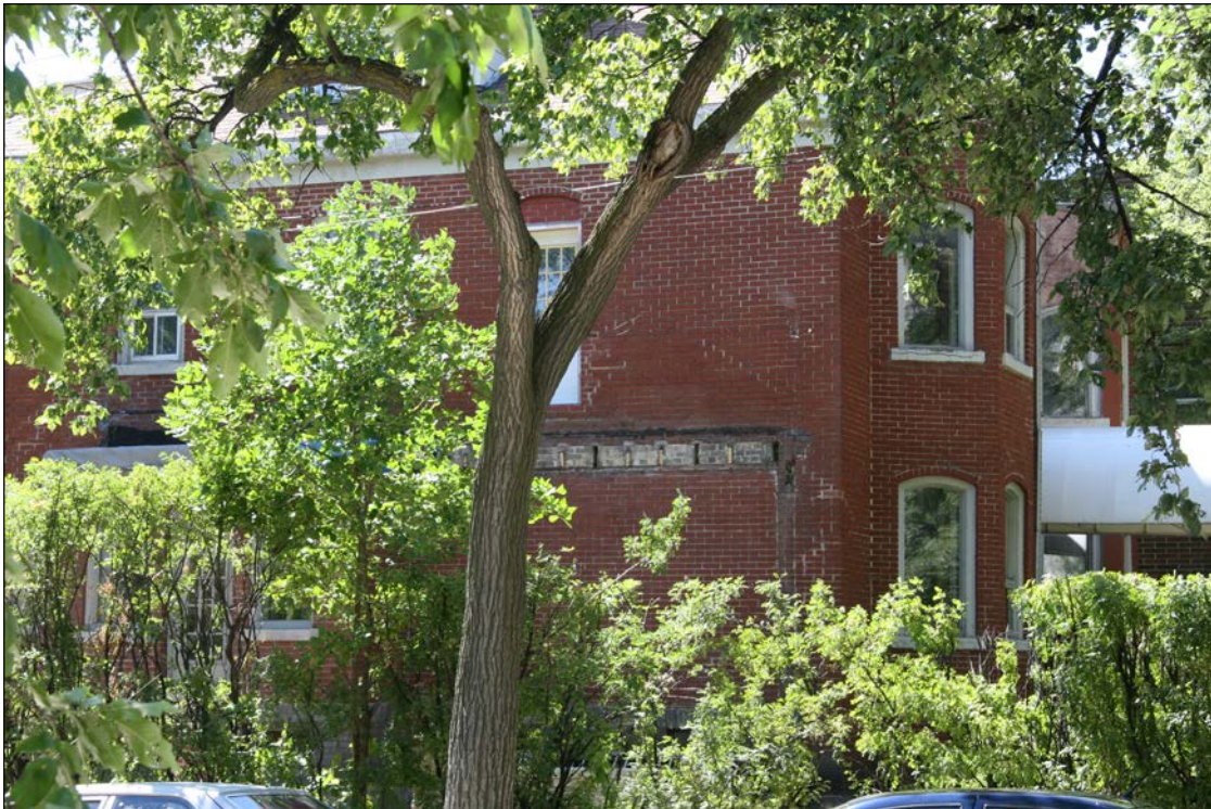
Plate 13 – John C. Falls House, 36 Roslyn Road, removal of east side porch, 2007. ( M. Peterson, 2007. )
