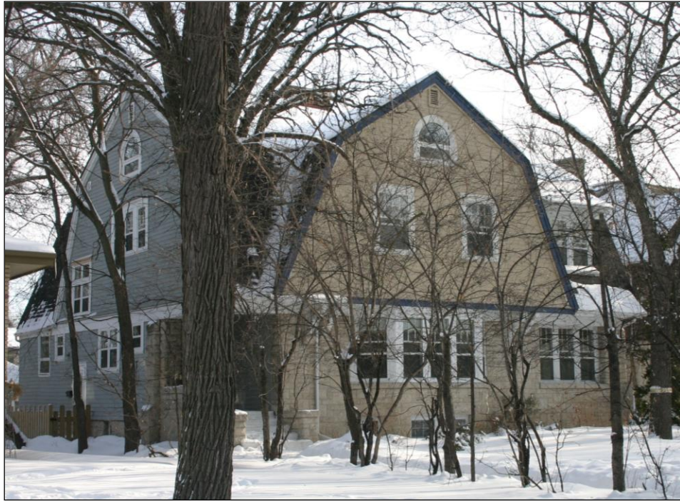
Front (west) and north façades, 2009
