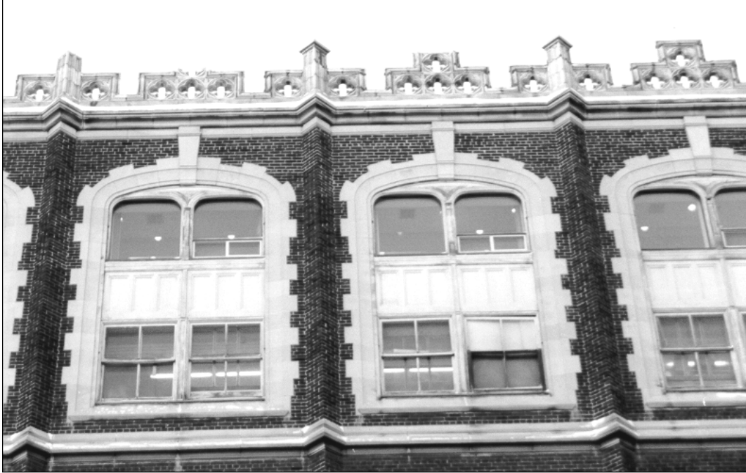
Plate 10 - Marlborough Hotel, portion of front (west) façade. (M. Peterson, 1998.)
