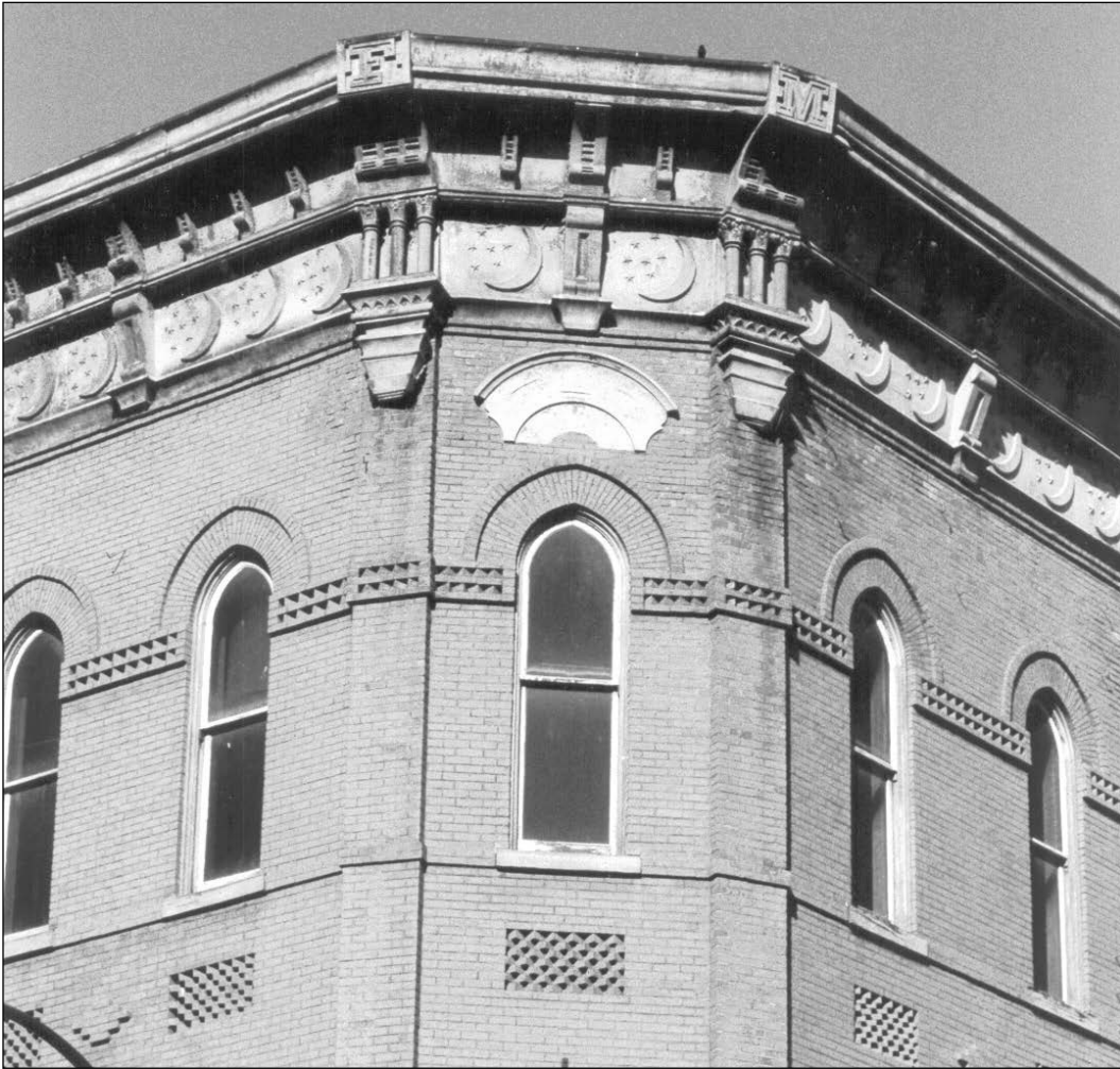
Plate 20 – Independent Order of Odd Fellows Building, 72-74 Princess Street, exterior detailing, date unknown. ( City of Winnipeg. )
