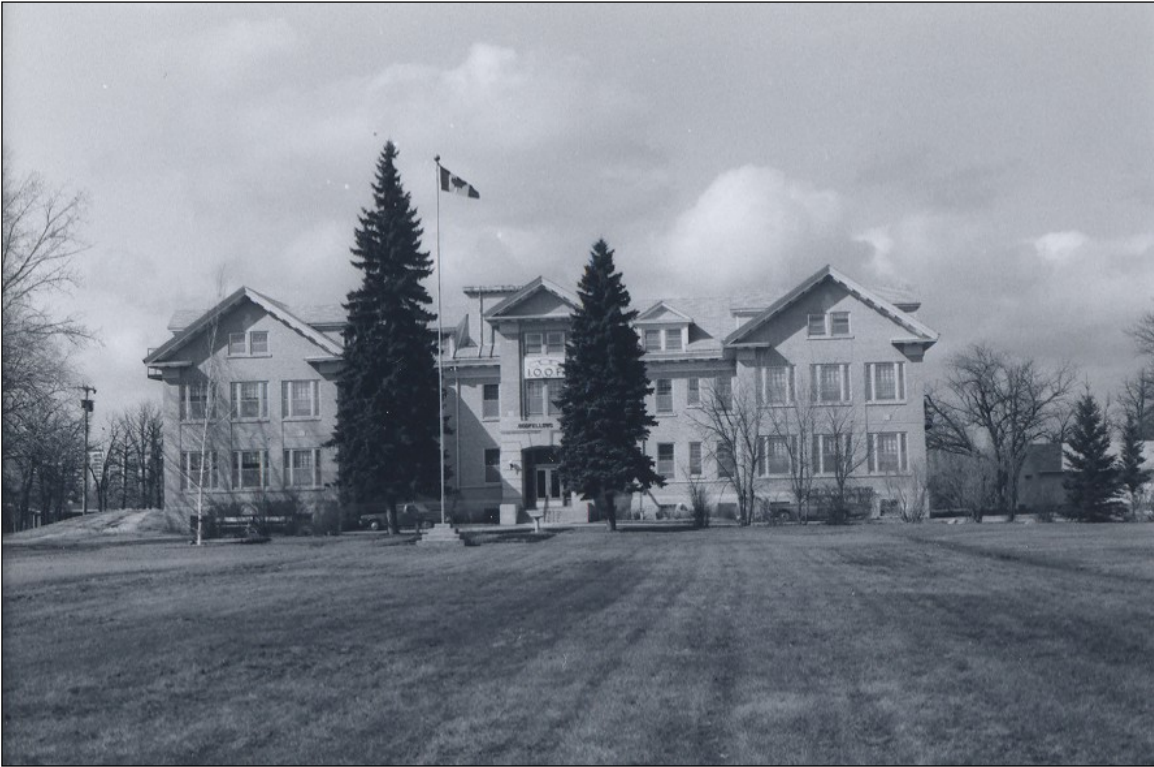
Plate 24 – Independent Order of Odd Fellows Home, 4025 Roblin Boulevard, front (south) façade, 1978; designed by J.H.G. Russell, built by S. Brynjolfsson, 1922. ( City of Winnipeg. )
